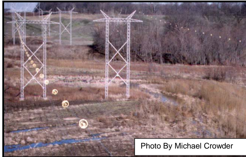
Photo 8 Swan Flight Diverters Installed at a 6-Meter Interval in Indiana
