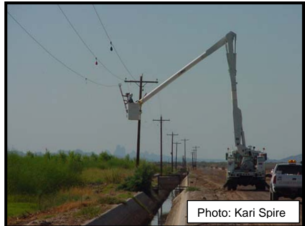
Photo 2 Flapper Installation
