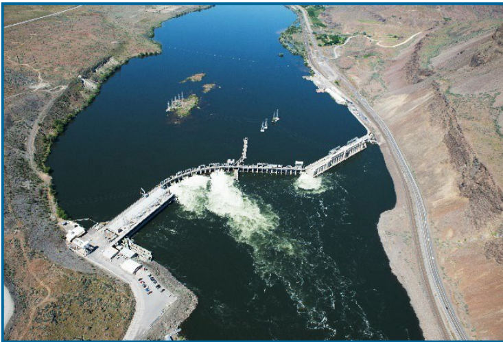
Aerial image of the Rock Island Hydroelectric Project.
