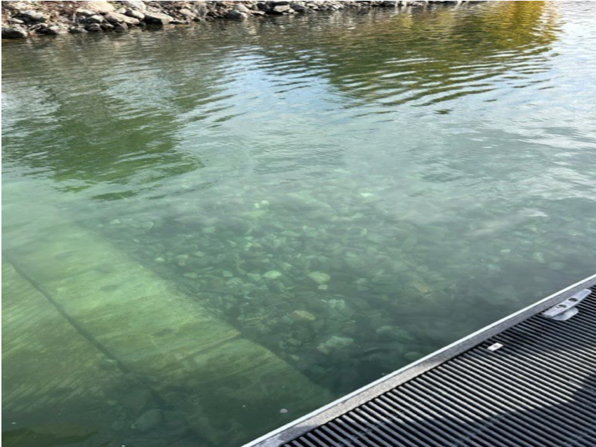
TEMPORARY FIX EXAMPLE
