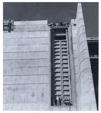
Photo 2: Looking upstream at the de-watered West fishway entrance during maintenance. In this photo the two gates are closed. (Archival Photo from Douglas PUD)
