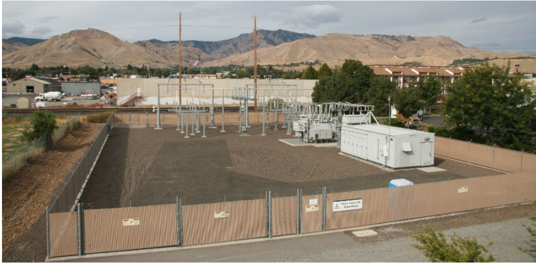
Walla Walla St. Substation
