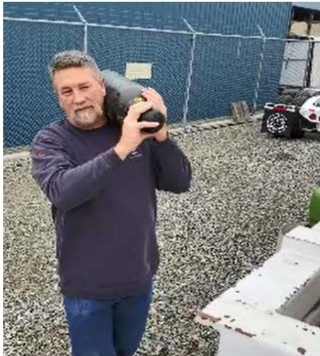
Smaller 35lbs replacement bottles easily moved and installed by 1 person. 2 bottles stored on mobile sub.
