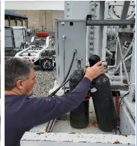
Smaller 35lbs replacement bottles easily moved and installed by 1 person. 2 bottles stored on mobile sub.
