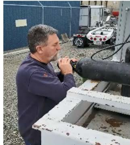
Smaller 35lbs replacement bottles easily moved and installed by 1 person. 2 bottles stored on mobile sub.
