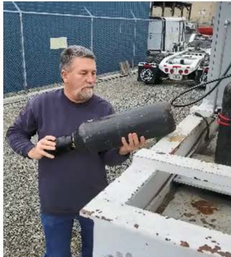
Smaller 35lbs replacement bottles easily moved and installed by 1 person. 2 bottles stored on mobile sub.
