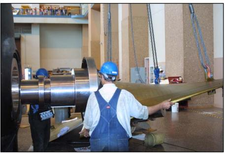
Requesting sole source approval for new seals and turbine bushings
