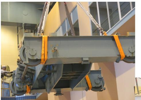
550 ton mobile cane picked off components through a hole in the roof
