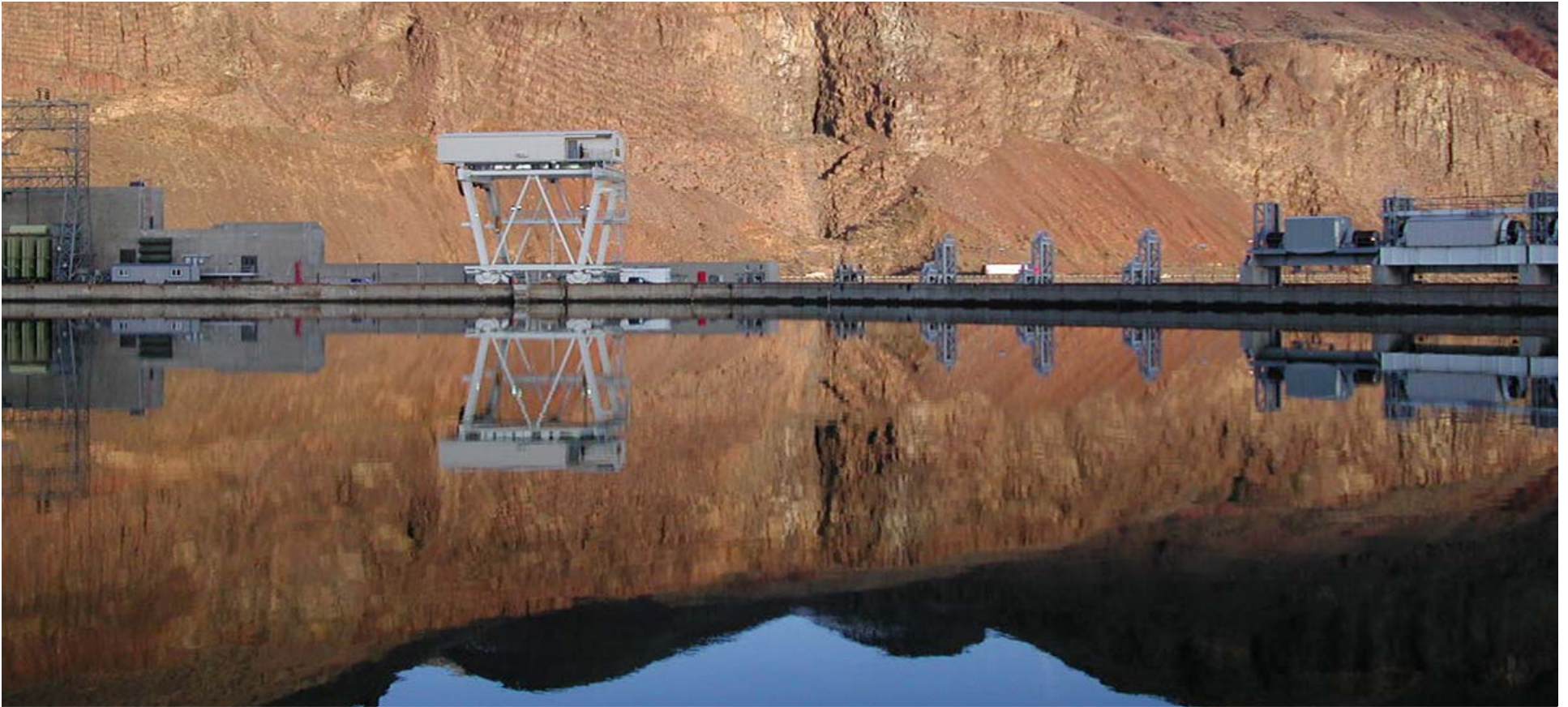
Rock Island Forebay
