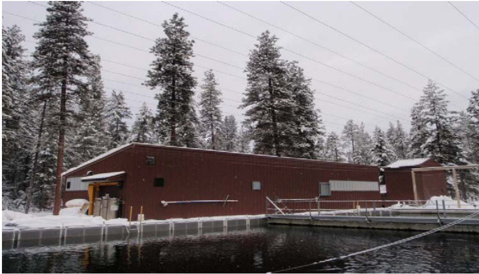
Chiwawa Acclimation Facility
