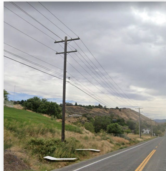
Double Circuit Distribution (Typical double circuit configuration)
