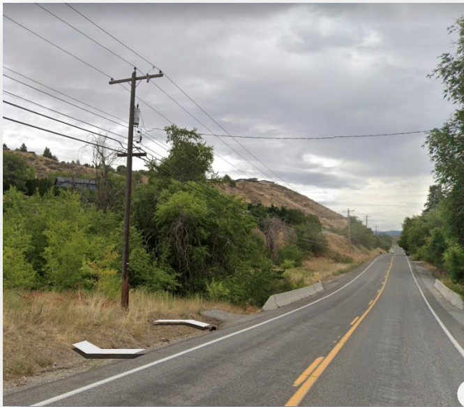
Single Circuit Distribution (Existing Mission Ridge Configuration)
