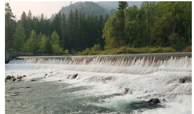
Tumwater Dam Spillway Repair $3.0M
