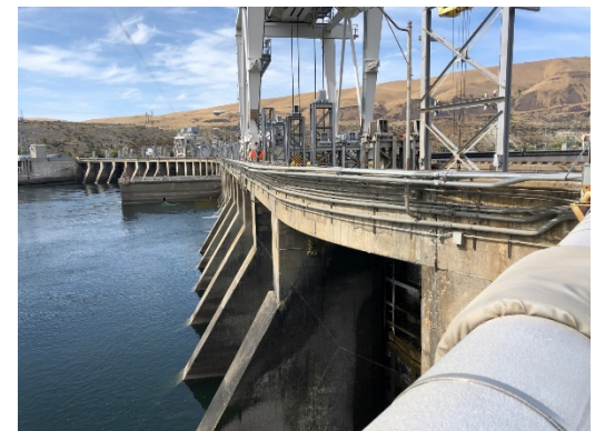
RI Spillway Pier Repair $2.6M
