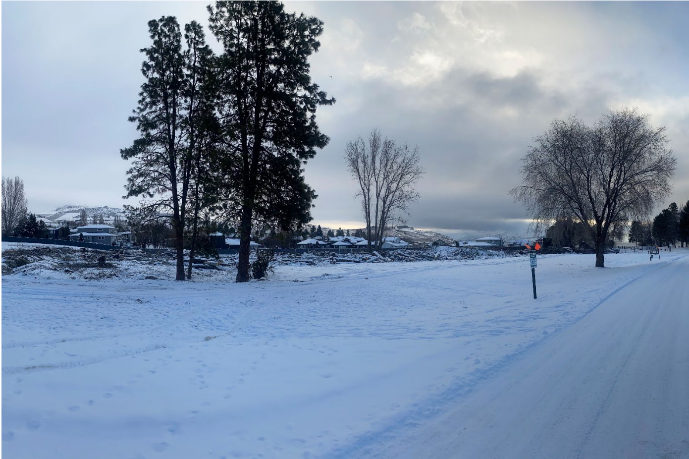
Area after tree/brush removal
