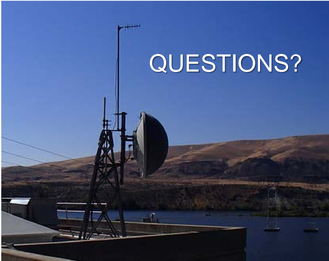
Rock Island Powerhouse 1 Microwave
