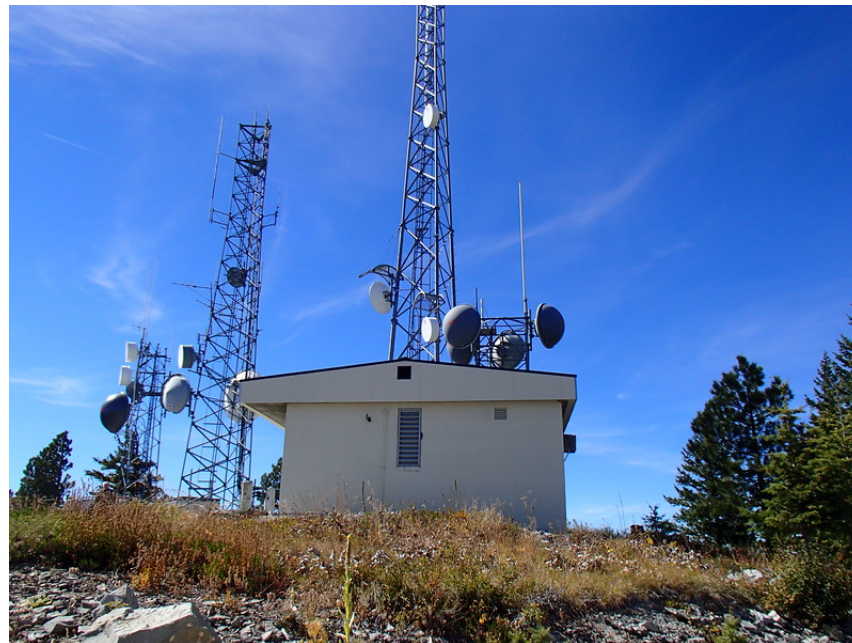
Burch Mountain Radio and Microwave Site
