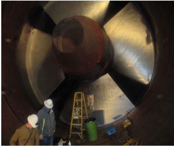
Rock Island PH2 Modernization Est. Completion: 2031 (all 8 units) 2022-2026: $238M
