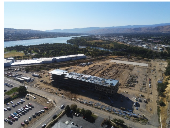
Operations/Service Center Est. Completion: Early 2023 2022-2023: $67M
