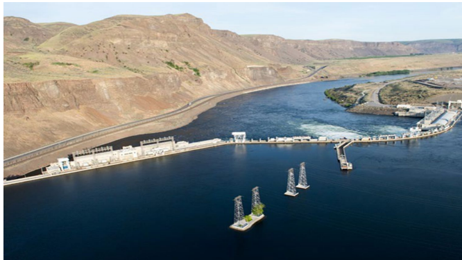
Rock Island PH1 Modernization Est. Completion: 2024 2022-2024: $52M
