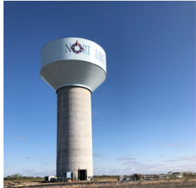
Composite Water Tower
