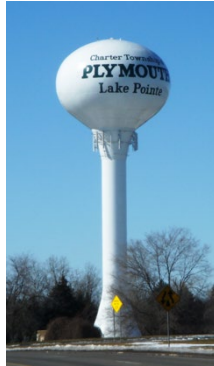
Single Pedestal Water Tower
