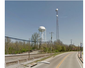
Structure with comms tower immediately next to it
