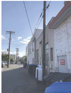
100 BLOCK EXISTING OVERHEAD UTILITIES (EAST) 2
