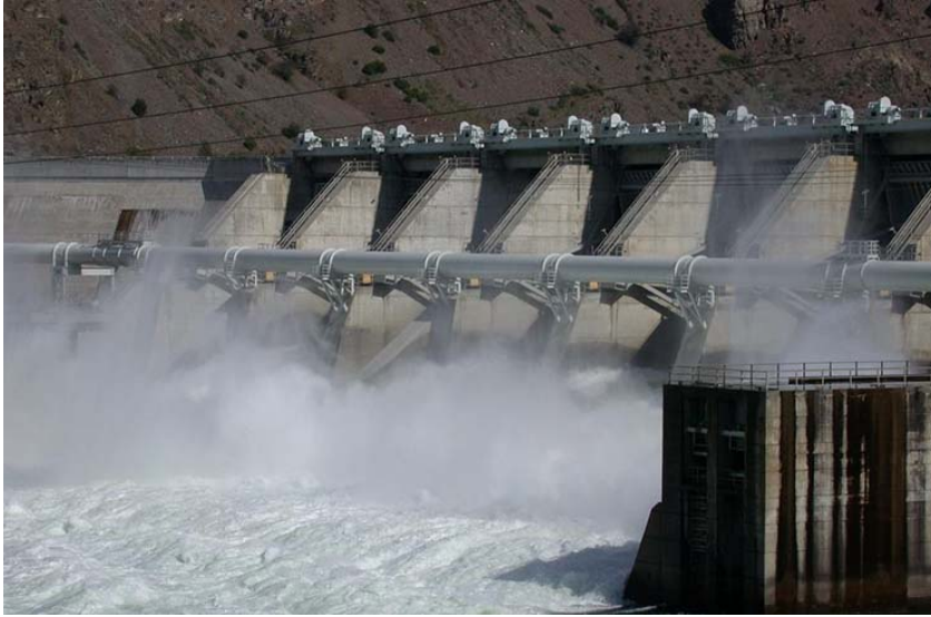
The Rocky Reach Dam, one of the dams on the Columbia River supplying cheap hydroelectric power to Chelan County, Washington. (Photo: Chelan PUD)
