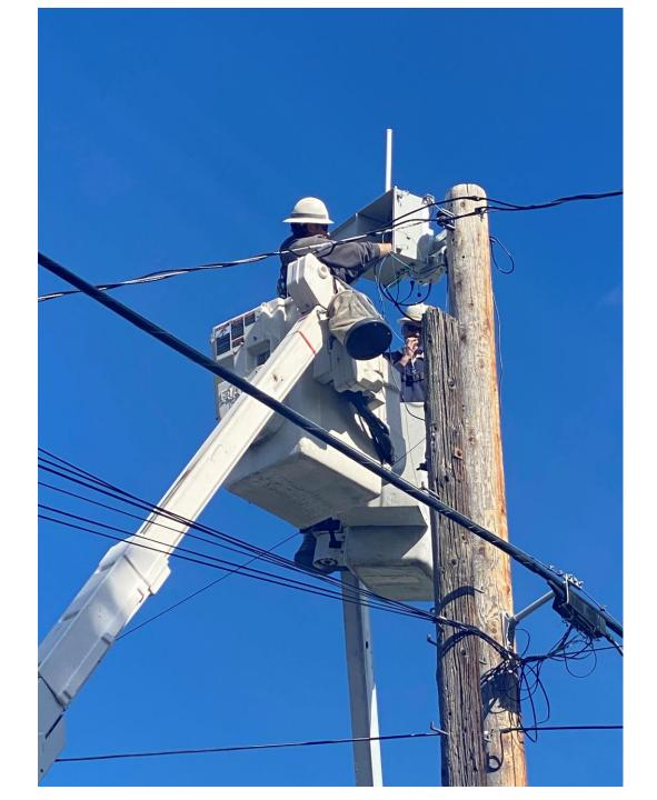
Tuesday April 26<sup>th</sup> CCPUD crews installed the first piece of aerial equipment to support the new Itron 2-way advanced metering network. This equipment, with several hundred AMI meters, will be activated as part of our beta testing phase prior to installing equipment and AMI meters county wide starting later this fall.
