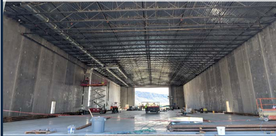
RI and RR facilities upgrades
