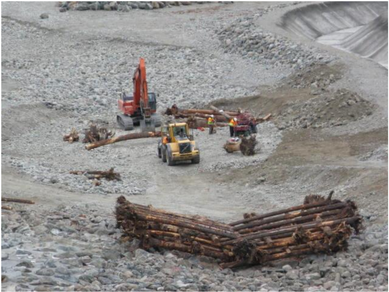
Picture taken on 12/1/08 looking south, showing the log jam at the entrance to the Habitat Channel. Forty-six trees, approximately 30 ft. long with root balls, make up this structure.
