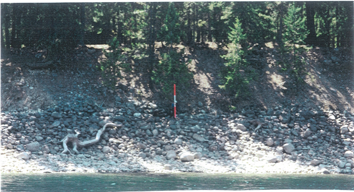
Site 26 Lucerne Campground Treatment area B (B = Double placed rock treatment, LWD, plantings) T3 contract spec. Photo CD 10 FR 50. Treatment length 33 feet
