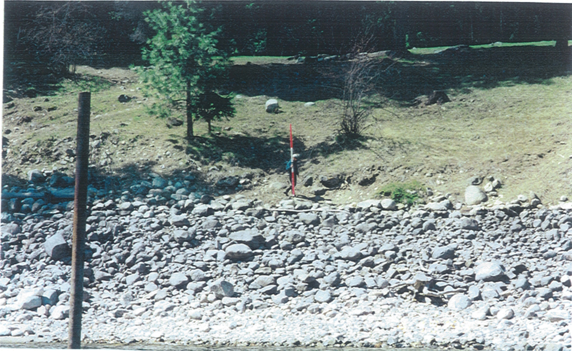
Site 25 Refrigerator Harbor Campground Treatment area B (Double Rock treatment, no LWD, no plantings) T3 modified contract spec. Photo CD 9 FR 58. Treatment covers 170 feet.
