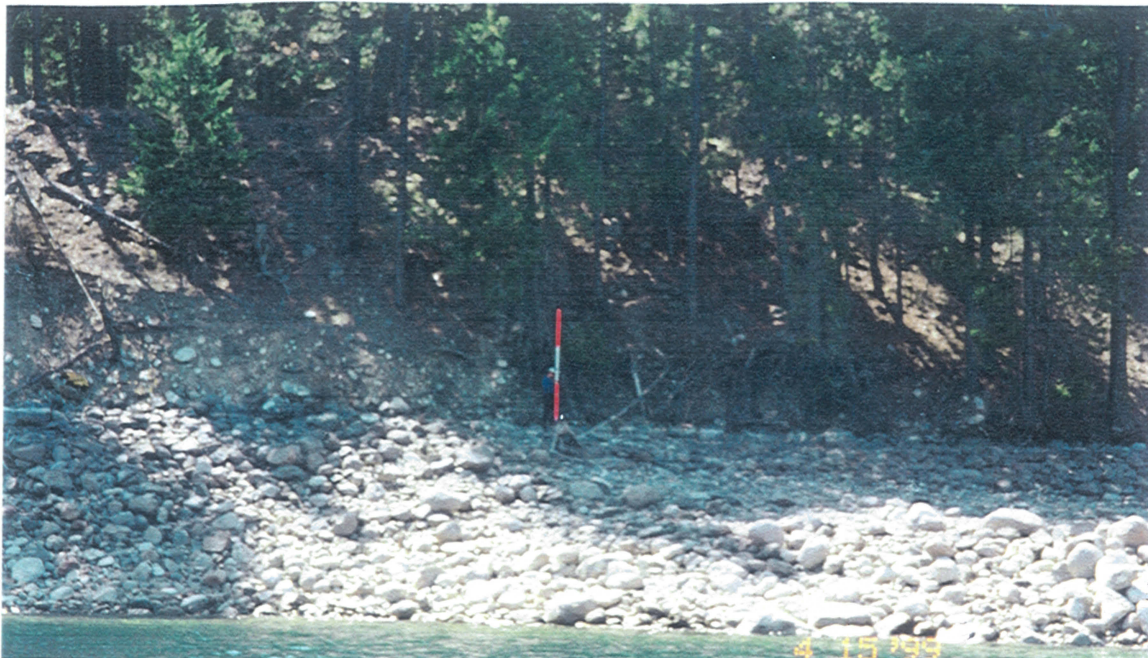
Site 26 Lucerne Campground Treatment area C (A =Enhanced placed rock treatment, LWD, plantings)T1 contract spec. Photo CD 10 FR 53.
