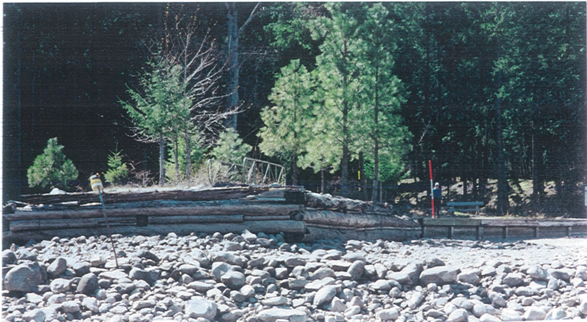
Site 26 Lucerne Campground Treatment area E (E=Enhanced placed rock treatment, no LWD or plantings, No wattles) TW contract spec CD10 Fr 56
