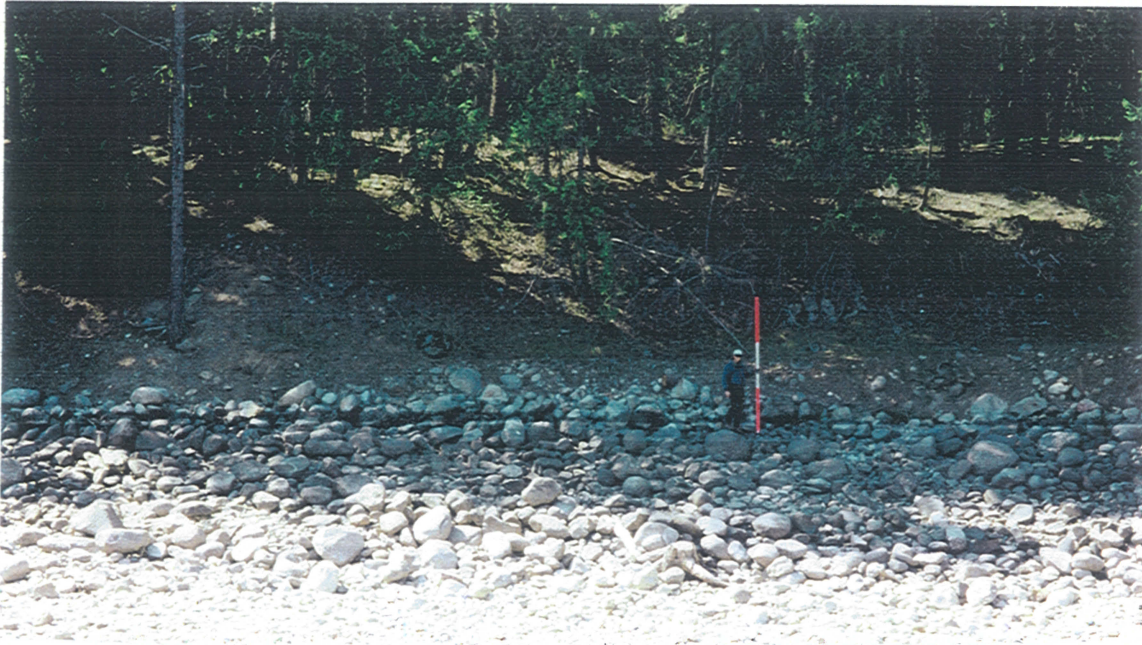
Site 25 Refrigerator Harbor Campground Treatment area's C/D (C=Enhanced placed rock treatment, LWD, plantings) T1 contract spec (D= Double rock treatment, LWD, plantings) T3 contract spec Photo CD 9 FR 66. Treatment D covers 57 feet.
