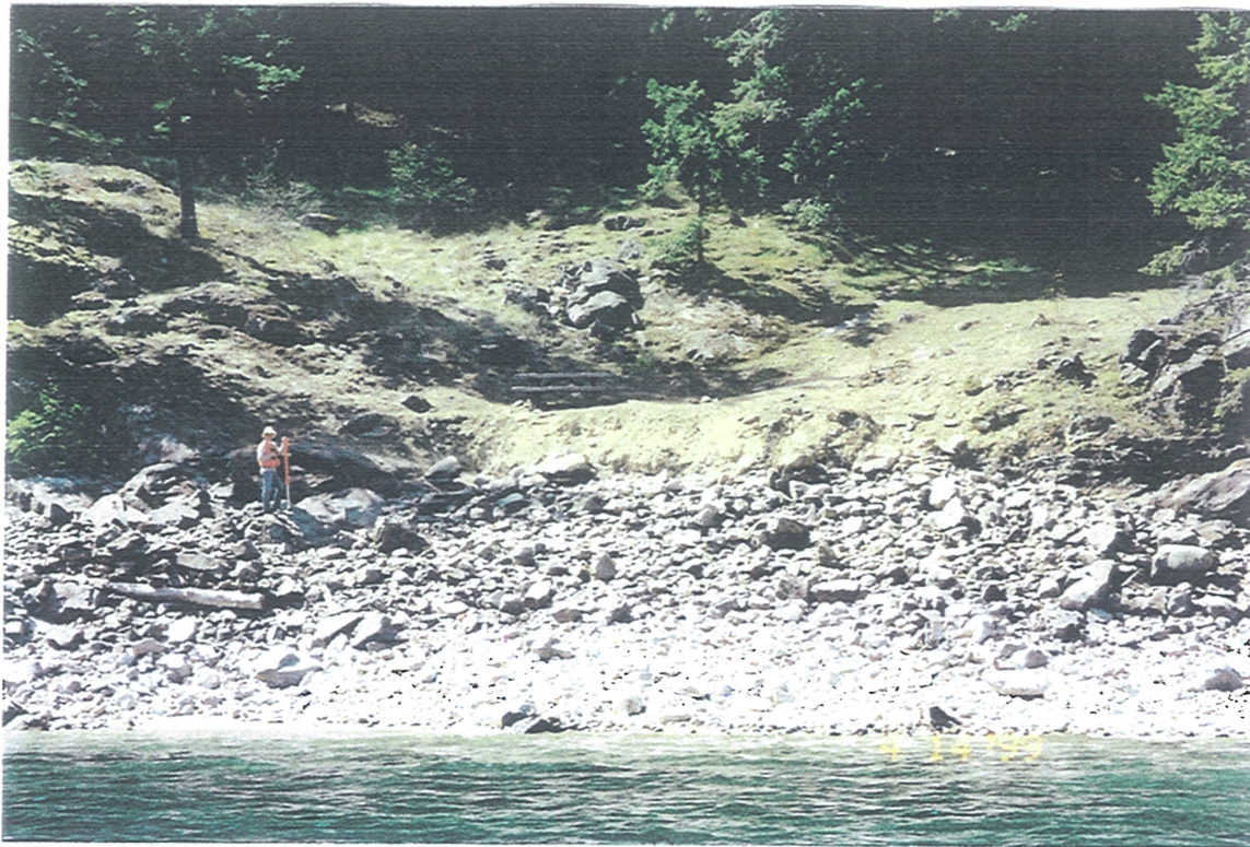
Site 24b Domke Falls Treatment area B (Enhanced placed rock no LWD, no plantings) T1 modified contract spec. Photo CD 6 FR 45
