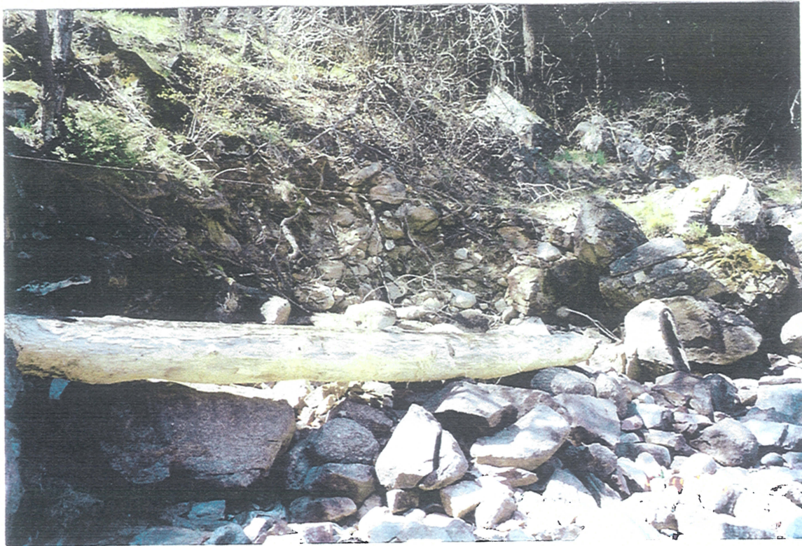
Site 24a Domke Falls Treatment area A (Enhanced placed rock, no plantings) T1 contract spec. Photo CD 10 FR 24
