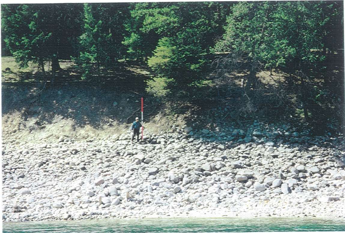
Site 25 Refrigerator Harbor Campground Treatment area C (Enhanced placed rock treatment, LWD, plantings) T1 contract spec Photo CD 9 FR 64. Treatment C covers 250 feet.
