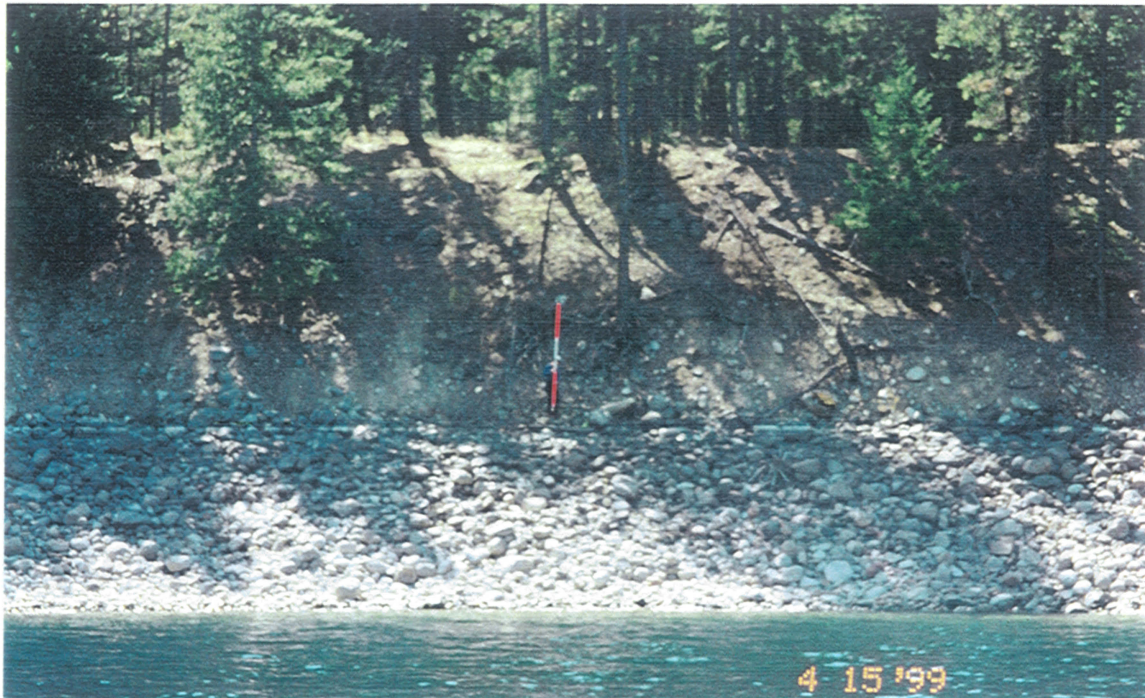
Site 26 Lucerne Campground Treatment area C (A=Enhanced placed rock treatment, LWD, plantings) T1 contract spec Photo CD 10 FR 52.
