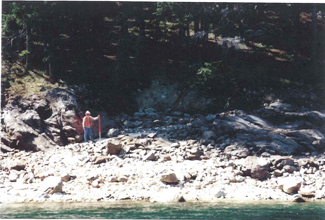
Site 24c Domke Falls Treatment area C (Enhanced placed rock, no LWD or plantings) T1 contract spec. Photo CD 6 FR 47.
