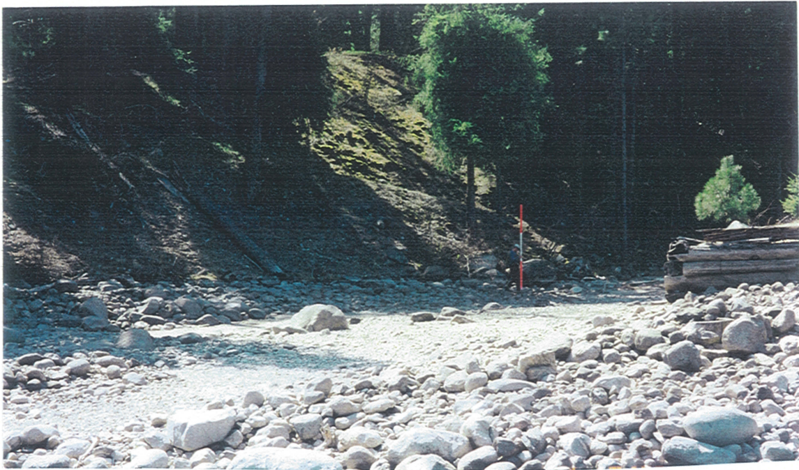
Site 26 Lucerne Campground Treatment area D (D= Scattered single and double rocks) T3 contract spec. Photo CD 10 FR 55.
