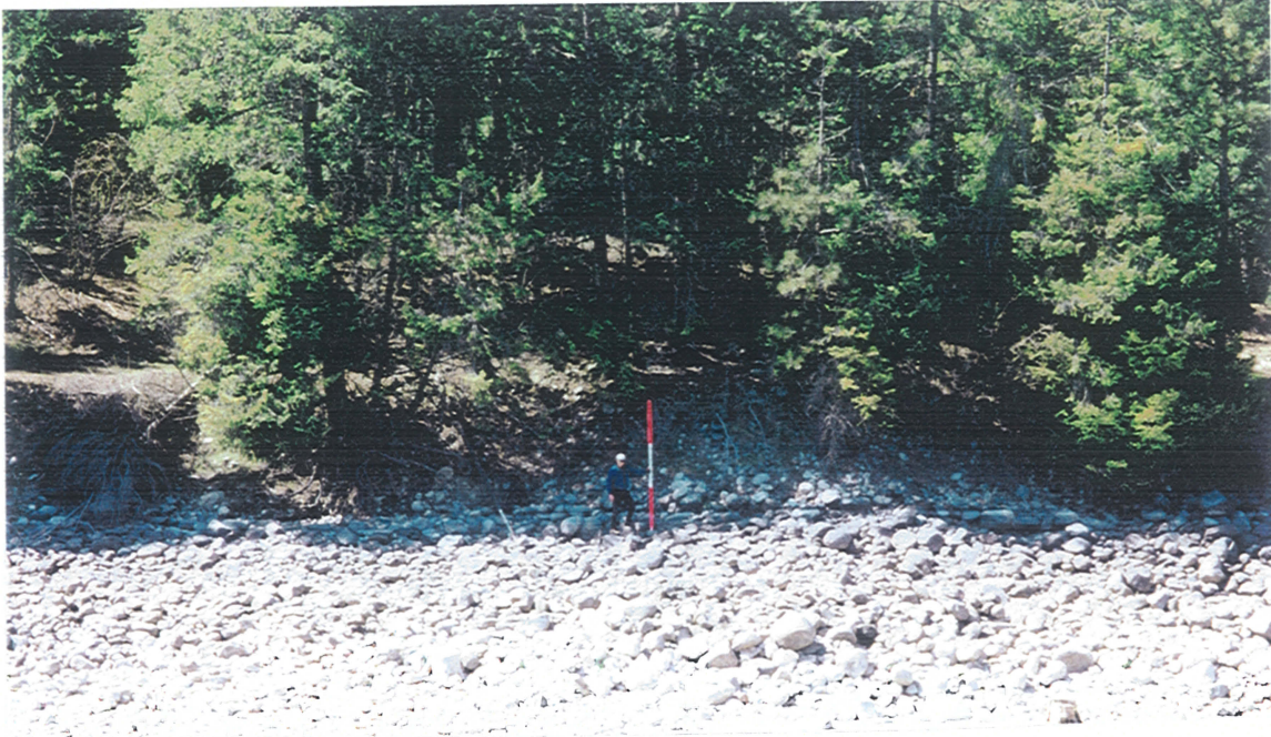
Site 25 Refrigerator Harbor Campground Treatment area E Ends. (Enhanced placed rock treatment, LWD, plantings) T1 contract spec. Photos CD 9 FR 71
