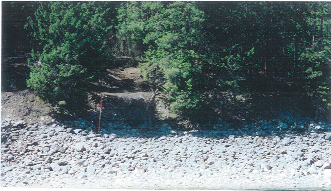
Site 25 Refrigerator Harbor Campground Treatment area E continued (Enhanced placed rock treatment, LWD, plantings) T1 contract spec Photos CD 9 FR 69
