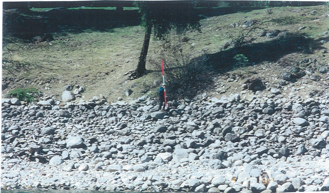
Site 25 Refrigerator Harbor Campground Treatment area B (Double Rock treatment, no LWD, no plantings) T3 modified contract spec. Photo CD 9 FR 59
