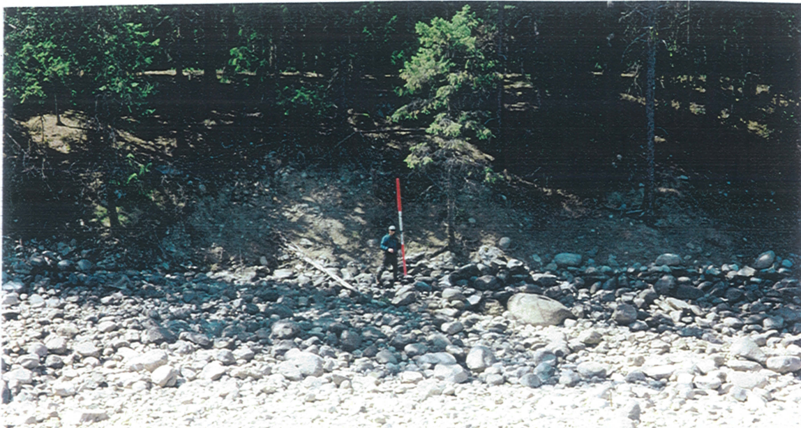
Site 25 Refrigerator Harbor Campground Treatment area C (Enhanced placed rock treatment, LWD, plantings) T1 contract spec Photo CD 9 FR 65.
