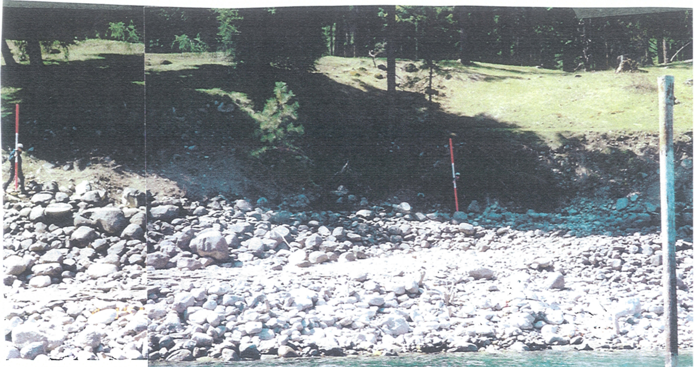
Site 25 Refrigerator Harbor Campground Treatment area B (Enhanced placed rock treatment, LWD, plantings) T1 contract spec Photo CD 9 FR 60 and 61
