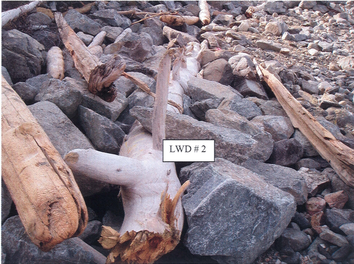
(Top view of LWD #2 pinned with rock)
