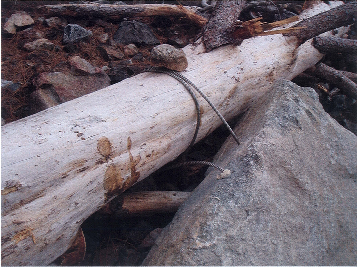
This is a close up photograph of LWD # 8 cabled with 1/2 inch stainless steel cable and glued with Hilti HY150 epoxy adhesive into drilled holes 8-9 inches deep.
