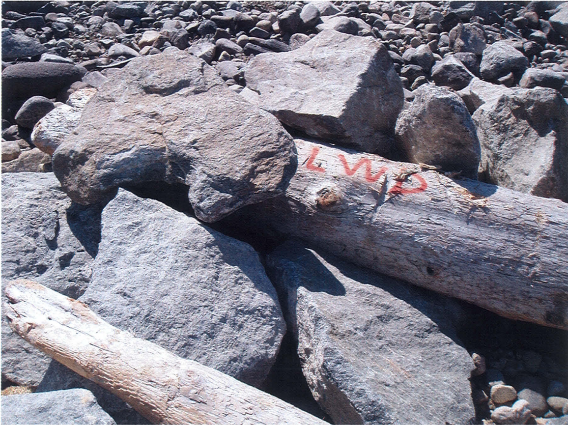
Upper end of LWD # 13 anchored with large single rock on top of LWD.
