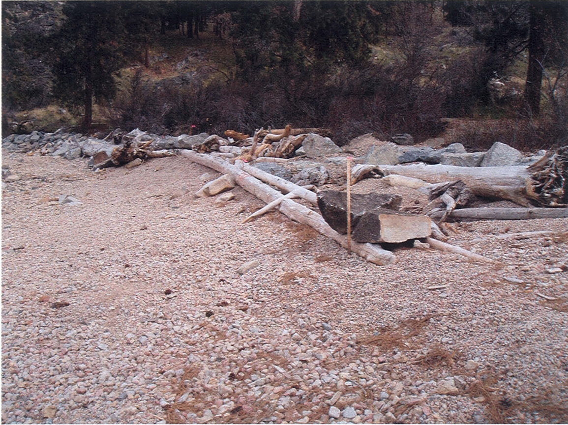
This shows LWD # 5 foreground with rock piles by end stakes, minor natural woody debris placed behind rock anchored pieces. Treatment B3 recreational steps are shown at the top of the stake.
