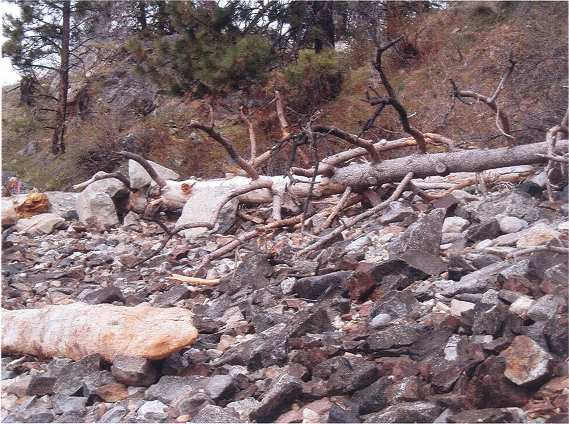
This is LWD # 8 it is anchored by cable and a large rock pile.
