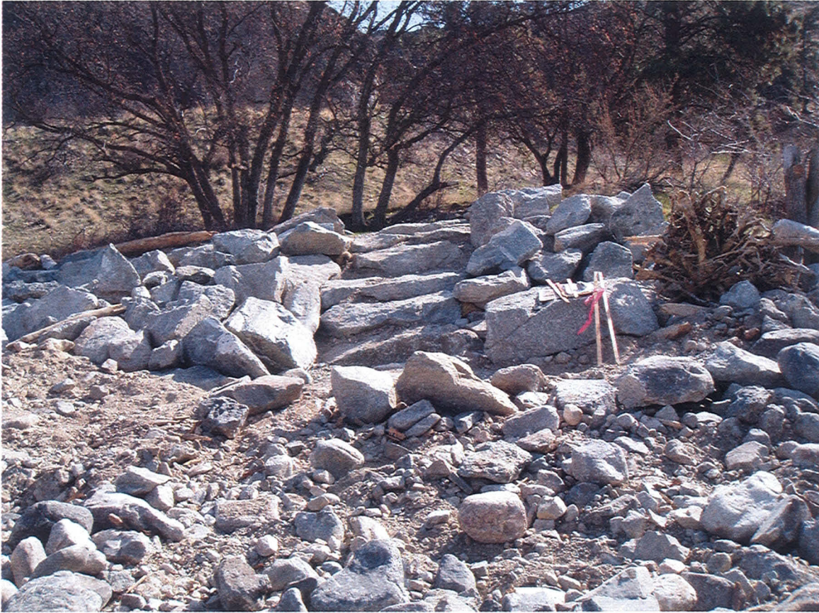
(Treatment B1) Rock steps for recreational access from shoreline camp site to water, treatment zone C1 ends at root wad right of the lathe and flagging. Large 4-5 foot relatively flat rock was used to create recreational access path.
