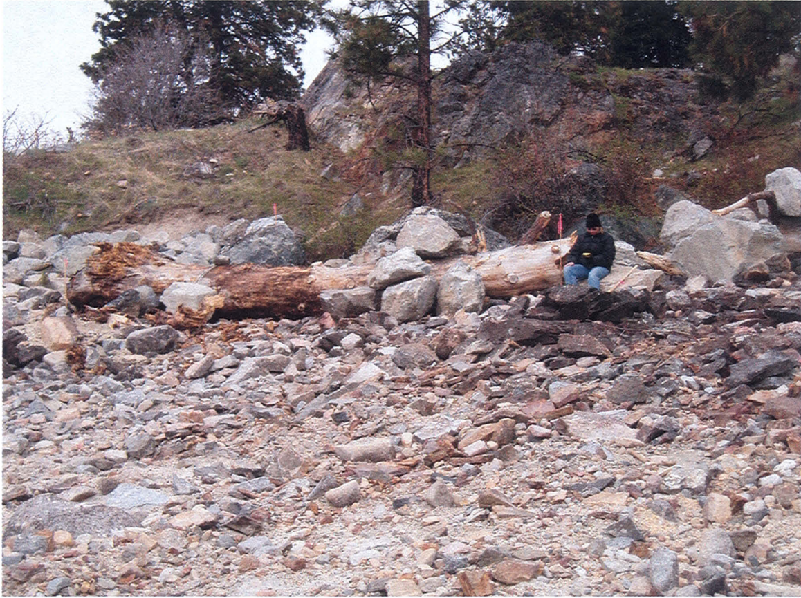
This is LWD # 7 in the foreground it is anchored with large rock and cabled wrapped. The left one-third of the picture shows the end of treatment zone A2. GPS point #7 is being collect by the person in the photograph.
