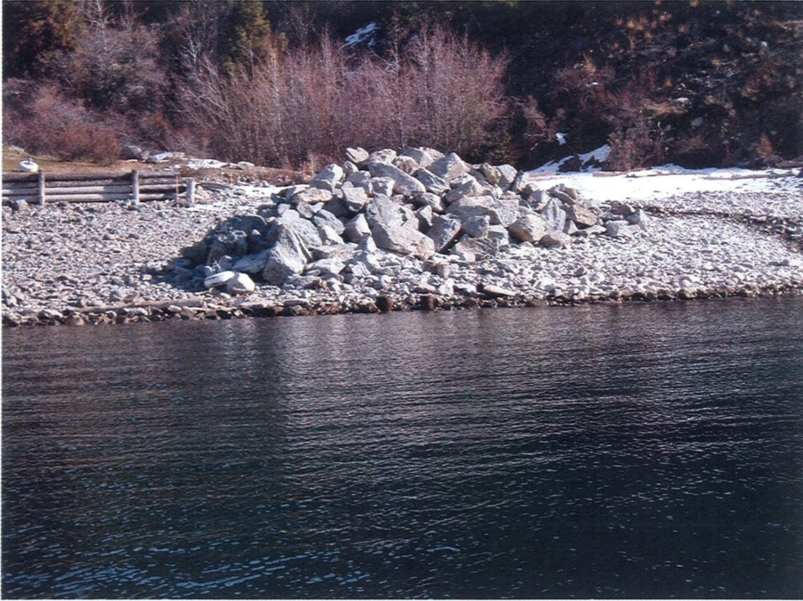
Approximately 190 tons of pre-placed rock for treatments D2 – E2, for treating 148 feet of erosion control repair. Note old crib wall and failed stream side section that has washed out.
