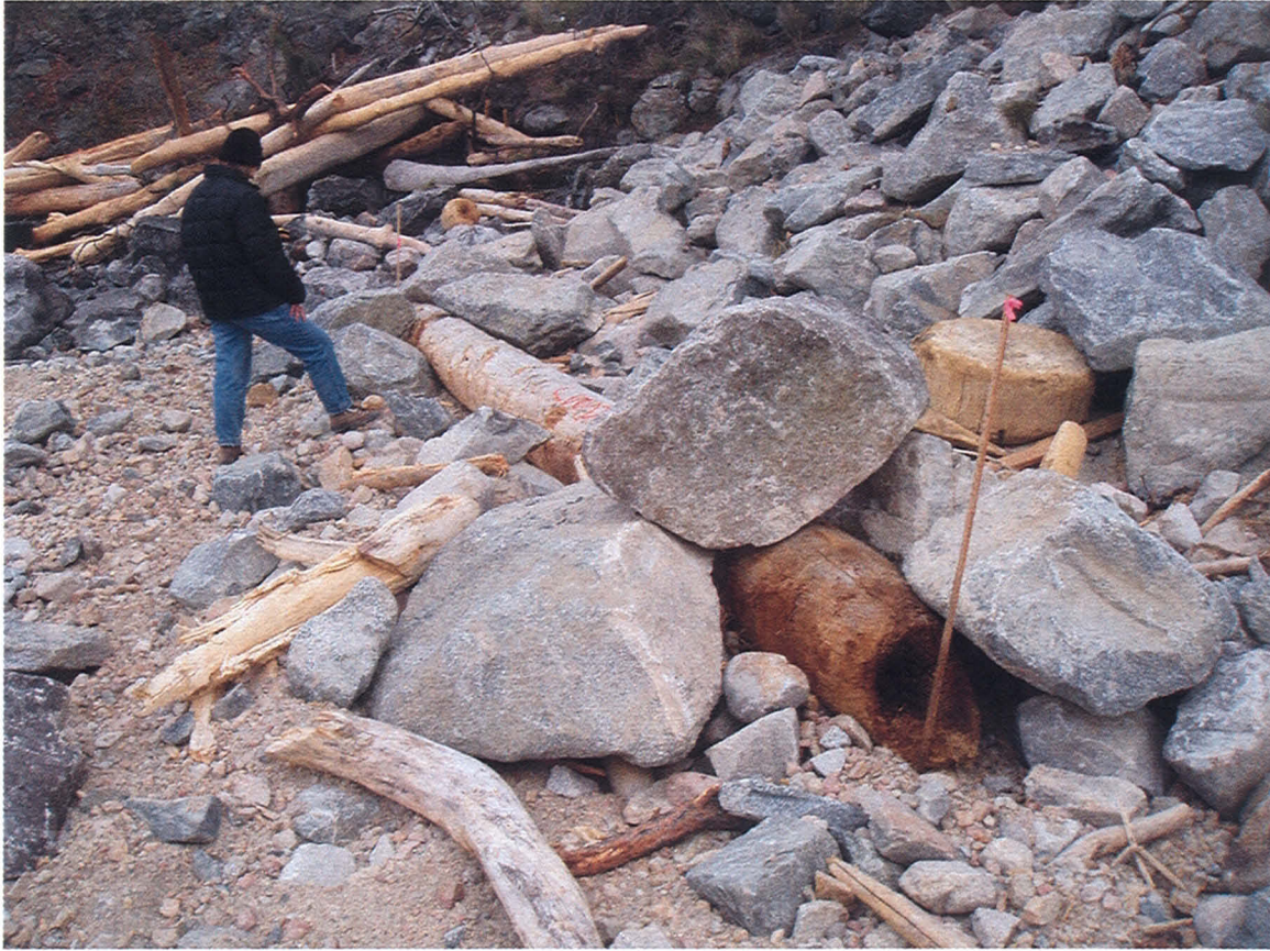
LWD #1 side view showing large rock piles used to anchor LWD. Natural smaller woody debris randomly piled left of treatment.
