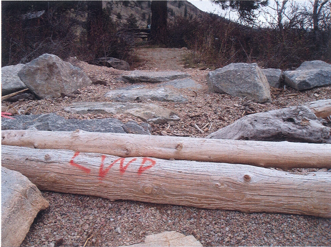
B3 recreational steps frontal view with LWD # 5, treatment right of steps changes to single rock placement with minor woody debris.
