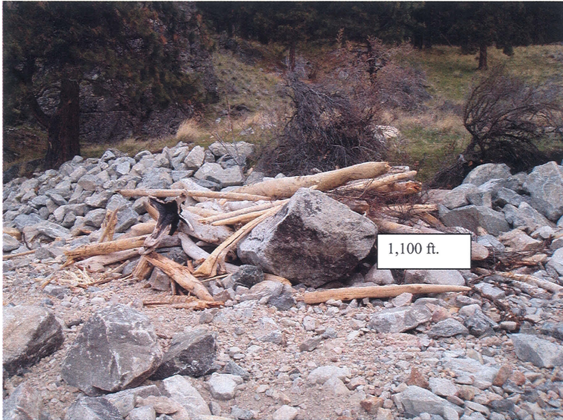
Minor area between treatments A1a and A1b approximately 12 feet of existing larger rock filled with minor woody debris from shoreline. Existing large rock shows approximate level of 1100 feet lake elevation.
