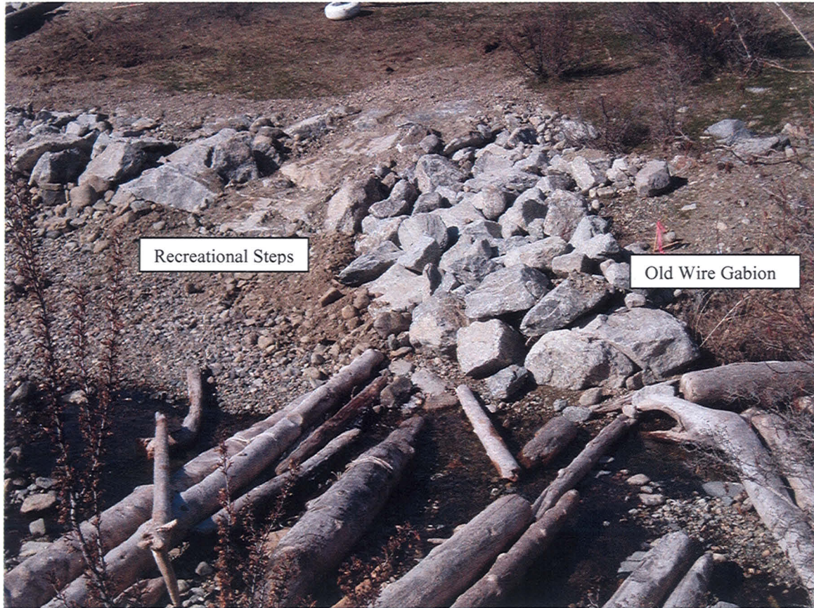
B5 are the recreational steps leading from Mitchell Shelter area to Lake and Mitchell Creek. Rock next to creek to pink flagged lathe is rock over the old exposed wire basket gabion from 1980's or 1970's repair when Mitchell Creek over flowed it channel.
