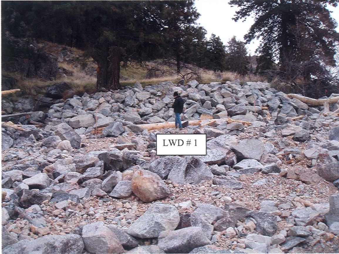
Start of treatment area A1a (50 feet) enhanced placed rock with LWD in foreground anchored with rock piles.
