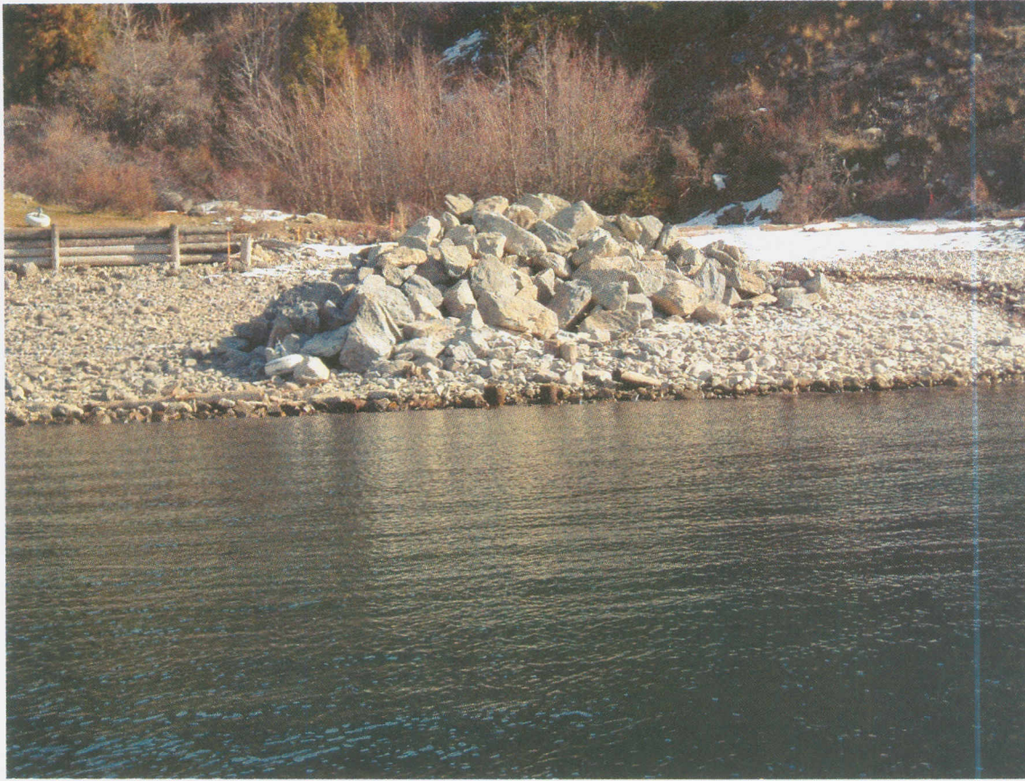
Approximately 190 tons of pre-placed rock for treatments D2 – E2, for treating 148 feet of erosion control repair.
