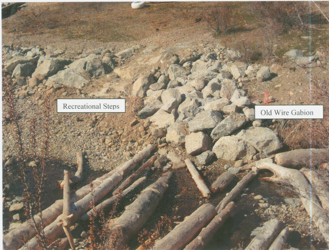
B5 recreational steps leading from Mitchell Shelter area to Lake Chelan and Mitchell Creek. Rock next to creek to pink flagged lathe is rock over exposed wire basket gabion from 1980's
