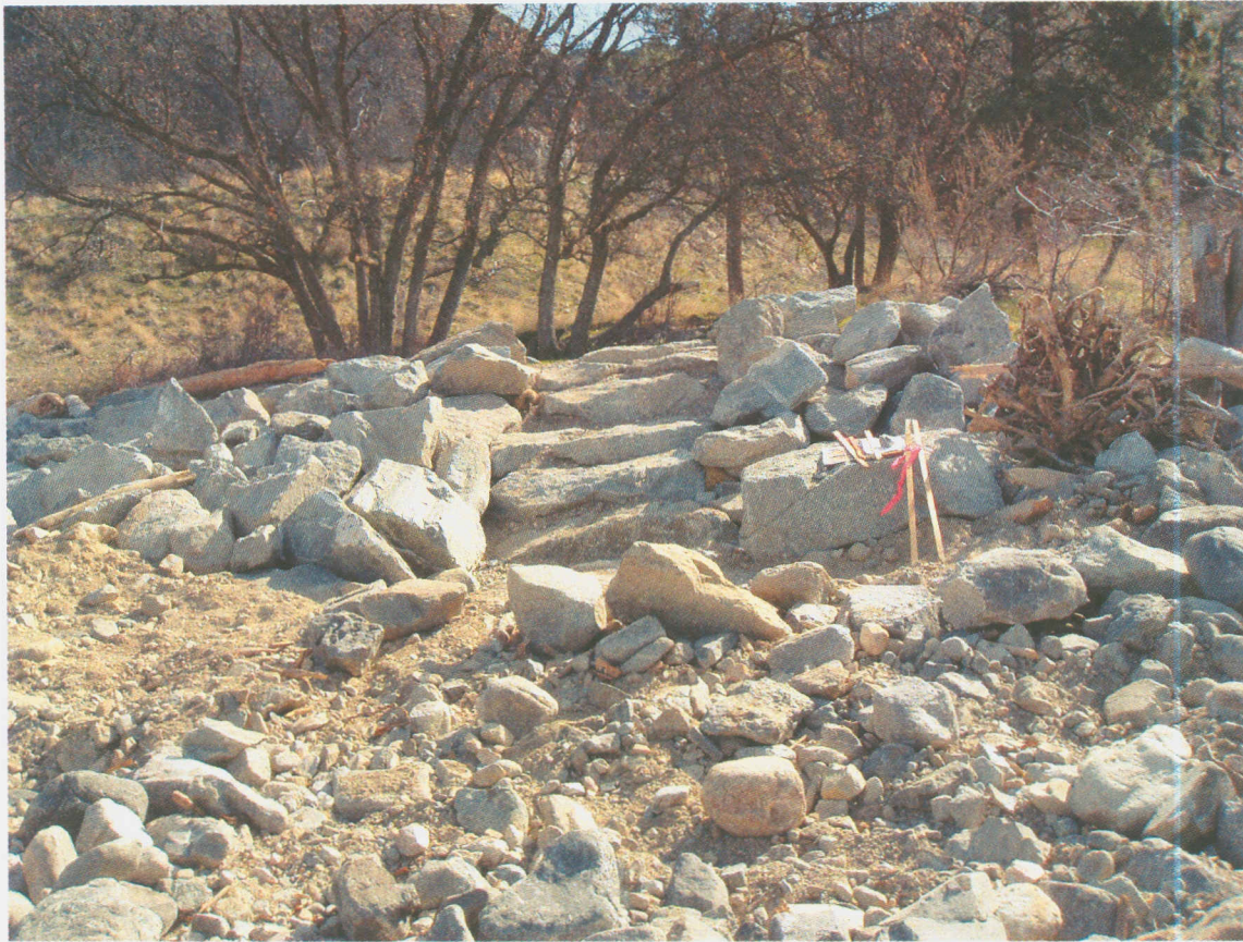
(Treatment B1) Rock steps for recreational access to water, treatment zone C1 ends at root wad right of the lathe and flagging. Large 4-5 foot relatively flat rock was used to create recreational access path.
