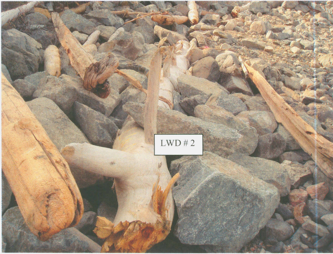
(Top view of LWD #2 pinned with rock)
