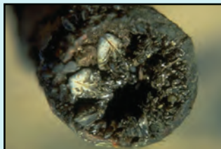
Zebra mussels blocking a pipe
