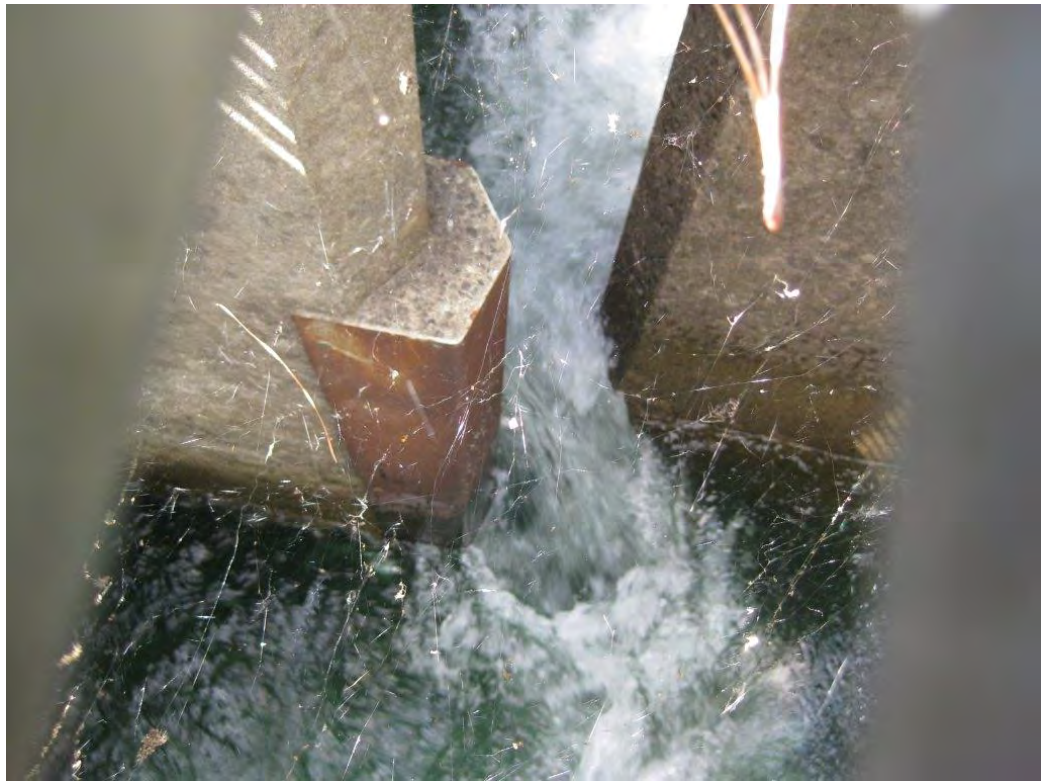
Figure 4. Fishway Vertical Slot, Modified from 15 to 12 inches Chelan PUD Tumwater Fishway Modifications
