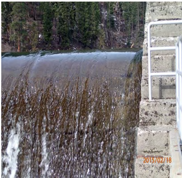
Figure 26 – Flow over dam ogee
