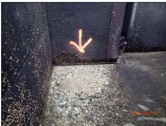
Figure 16- Sediment and gravel accumulations downstream of slot stub walls
