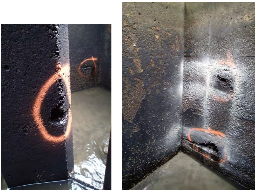
Figure 14 and Figure 15. Spalling concrete in slot surface and pool sidewall corner of Tumwater Dam fish ladder
