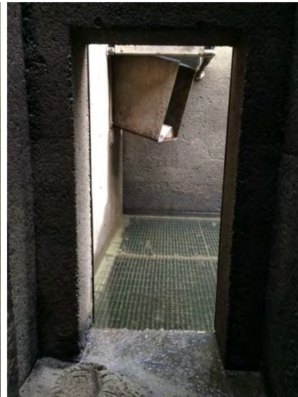
Figure 24. Floor screens and steep-pass
