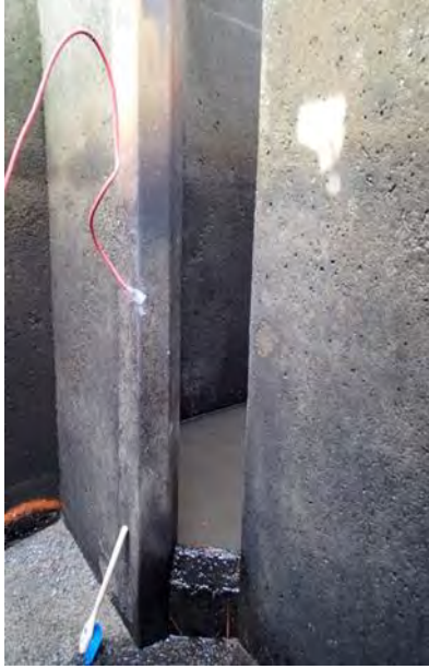
Figure 10. Sill at base of typical Tumwater Dam fish ladder slot
