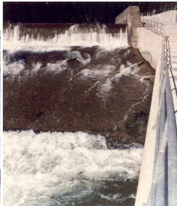
Figure 27 – Concrete apron, ogee in background
