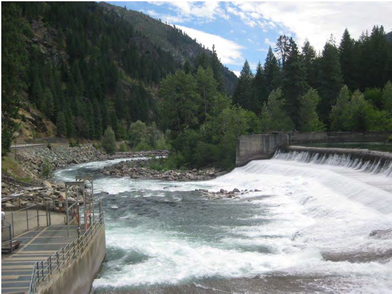
Figure 1. Fishway Entrance, Right Abutment and Tailwater Chelan PUD Tumwater Fishway Modifications
