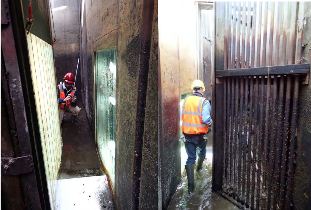
Figure 11 and Figure 12. Counting window and upstream picket lead crowder.
