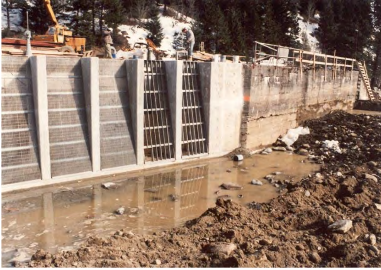
Figure 19. Tumwater AWS and lower ladder trash racks
