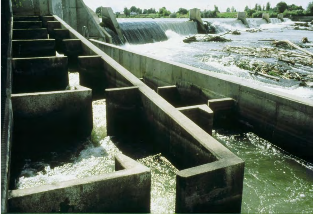
Figure 7. Example of vertical slot ladder pool and slot flow hydraulic conditions – note pools include both aerated turbulent flow near the slot jet, and lower turbulence, green water further from the jet
