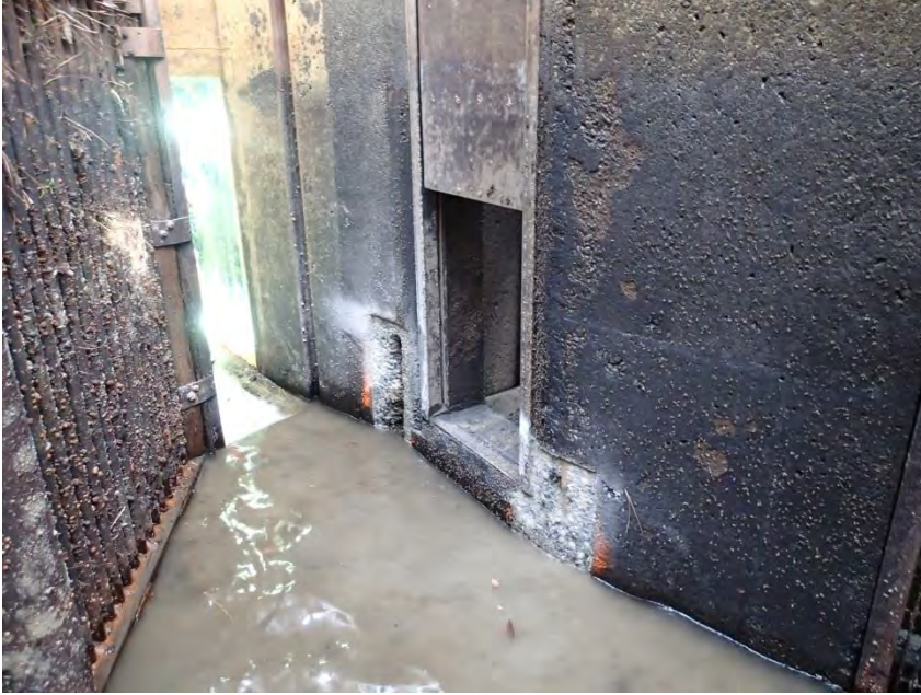
Figure 13 – Upstream-looking view of picket leads, counting window, and emergency trap adult return port (with gate in upward and open position)
