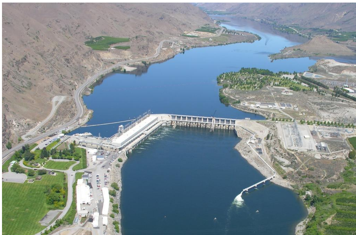
Figure 2. Rocky Reach Dam.
