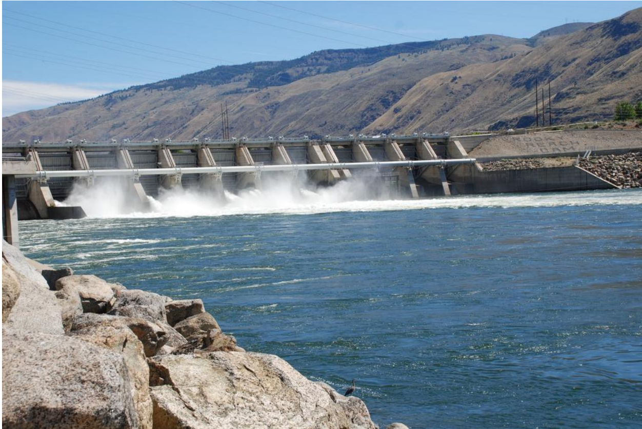
Figure 3. Rocky Reach Project spillways.
