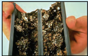
Zebra mussels in a cut-away pipe
