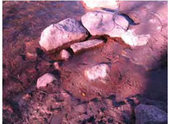
View of outlet at base flow.
