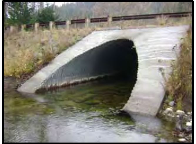
Nason Creek culvert inlet.
