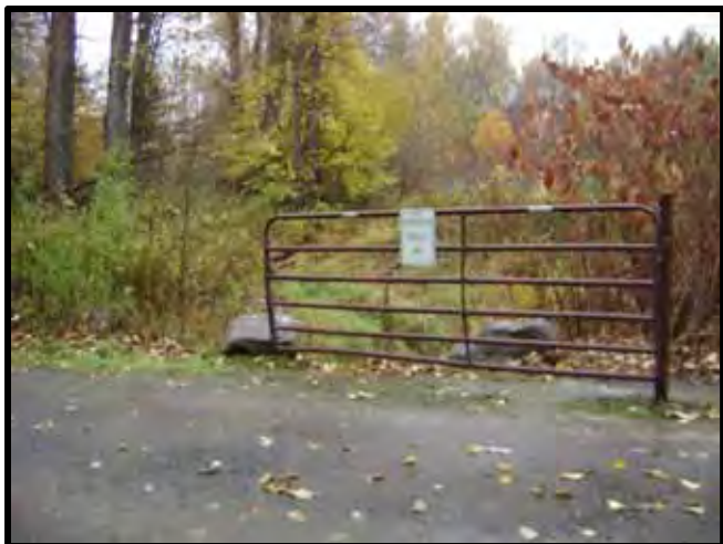
Trail where culvert crosses.
