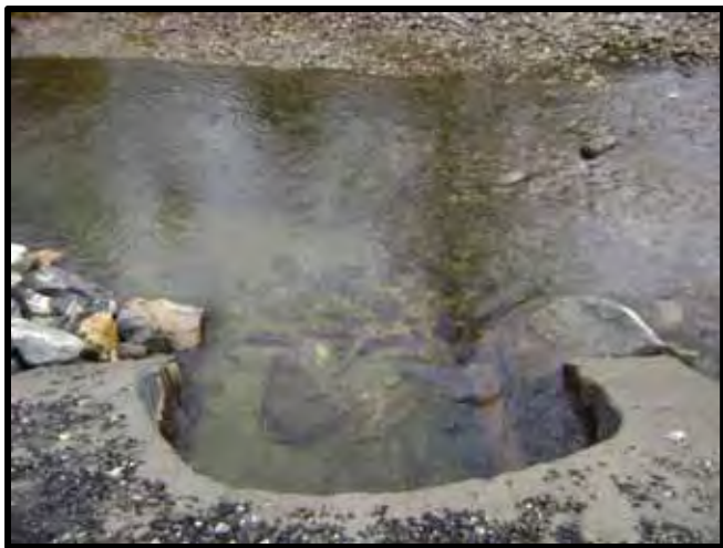
Nason Creek at oxbow inlet culvert.
