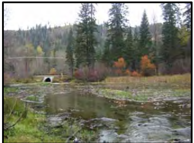
Looking back at inlet culvert.
