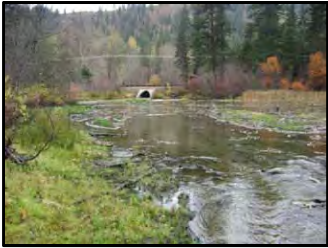
Looking back at inlet culvert (2).
