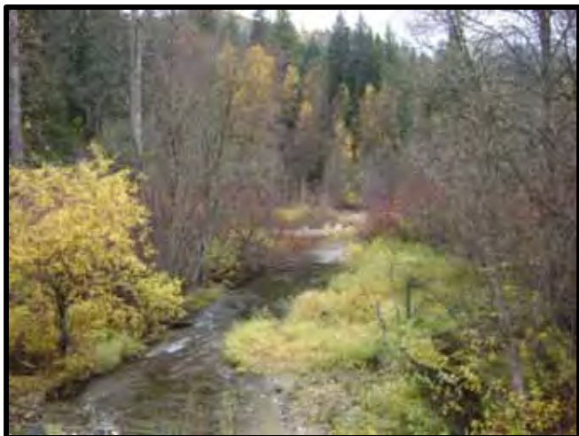
Outlet downstream of culvert.
