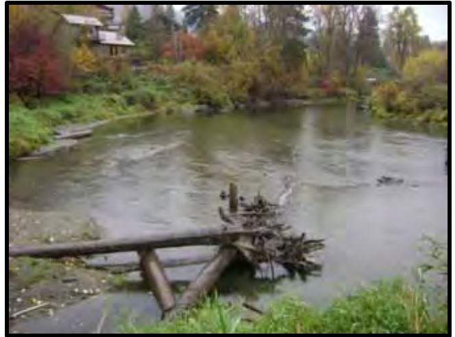
Outlet and Wenatchee side channel.
