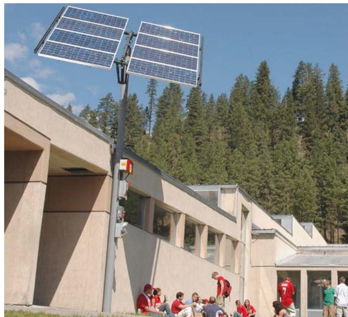
*Panels at Cascade High School, Leavenworth, are mounted onto a tracking device that follows the sun's movement.*
