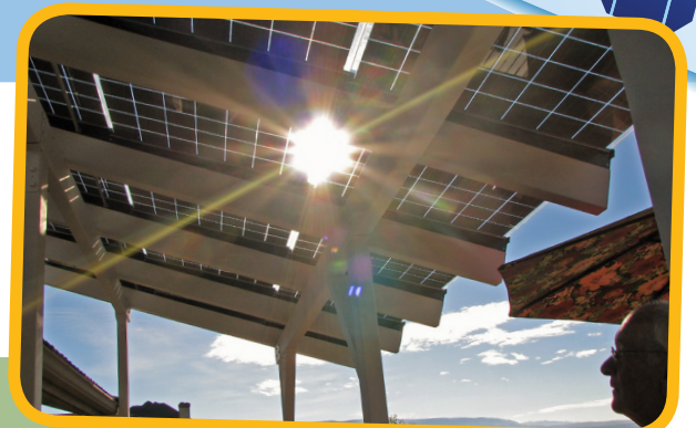
Right: Twenty-four modules form a canopy over the deck at Jim and Lynn Brown's home in Wenatchee.
