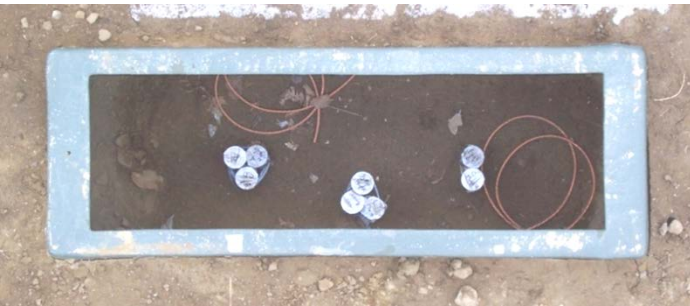
THREE PHASE TERMINATION CABINET INSTALLATION - Figure 13 (Backfilled, with ground tails into cabinet)
