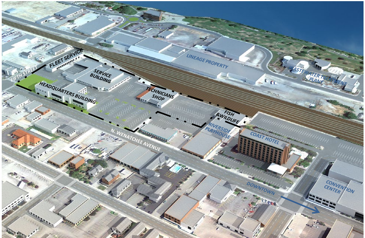
View of site area along Wenatchee Avenue.
