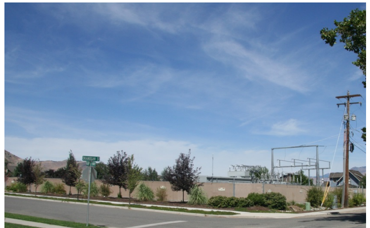
Okanogan Substation (Wenatchee)
