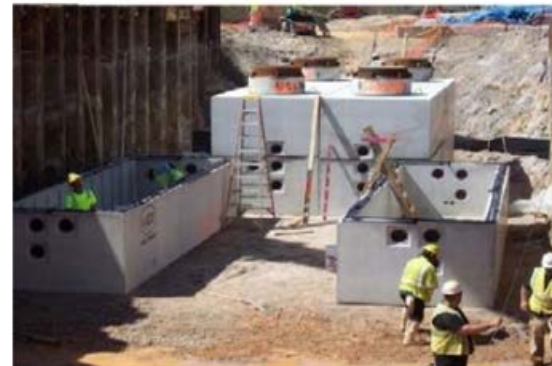
Figure 18-15 Vault Placement
