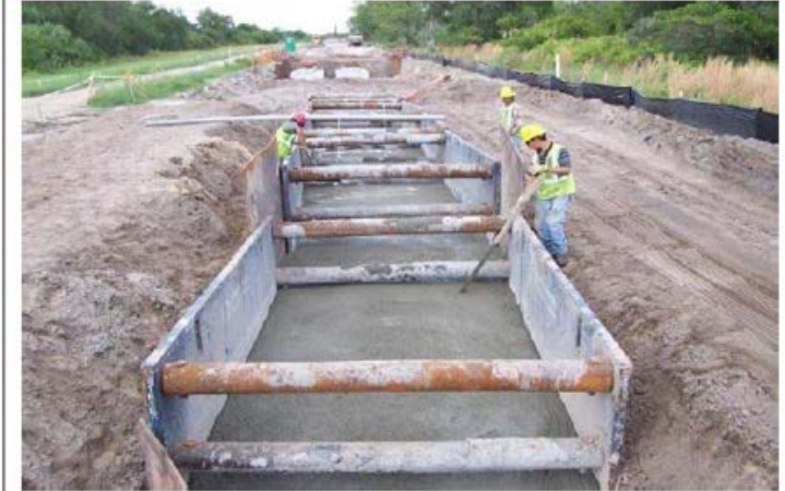
Figure 18-14 Conduit Backfilling
