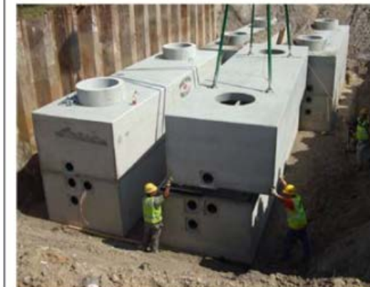
Figure 18-16 Vault Placement - Top
