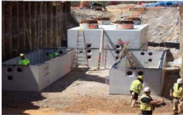
Figure 18-15 Vault Placement
