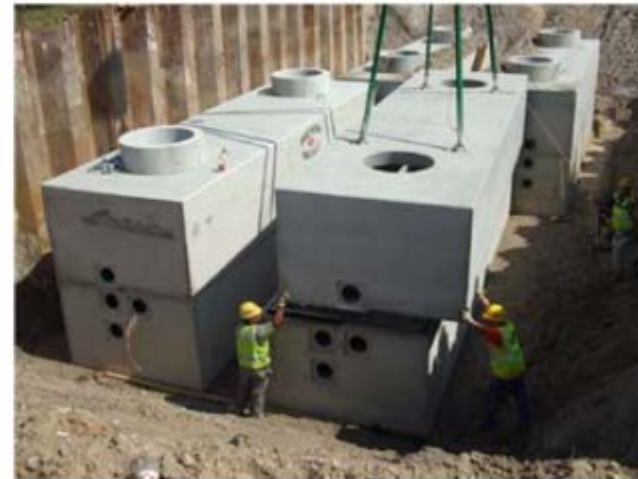
Figure 18-16 Vault Placement - Top
