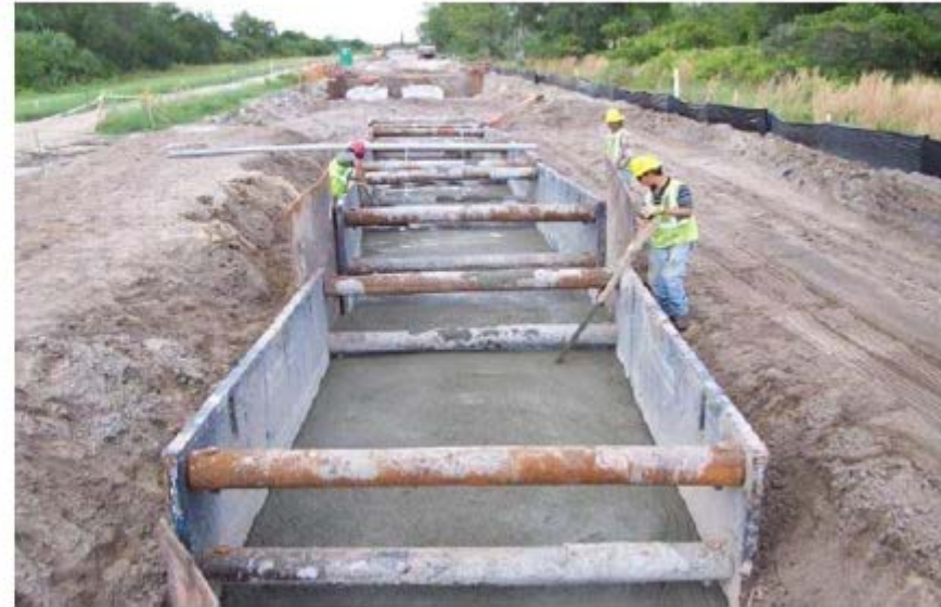
Figure 18-14 Conduit Backfilling
