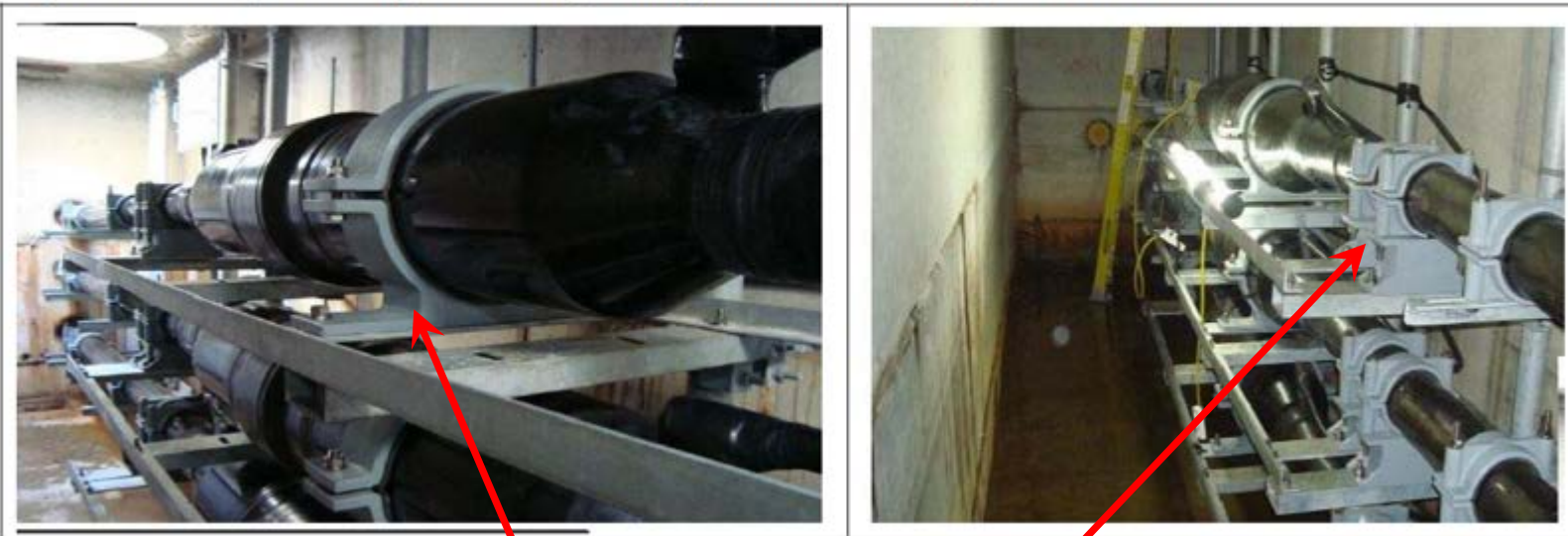
Figure 16-1 Rigid Straight-Through Single Circuit Arrangement in Vault
