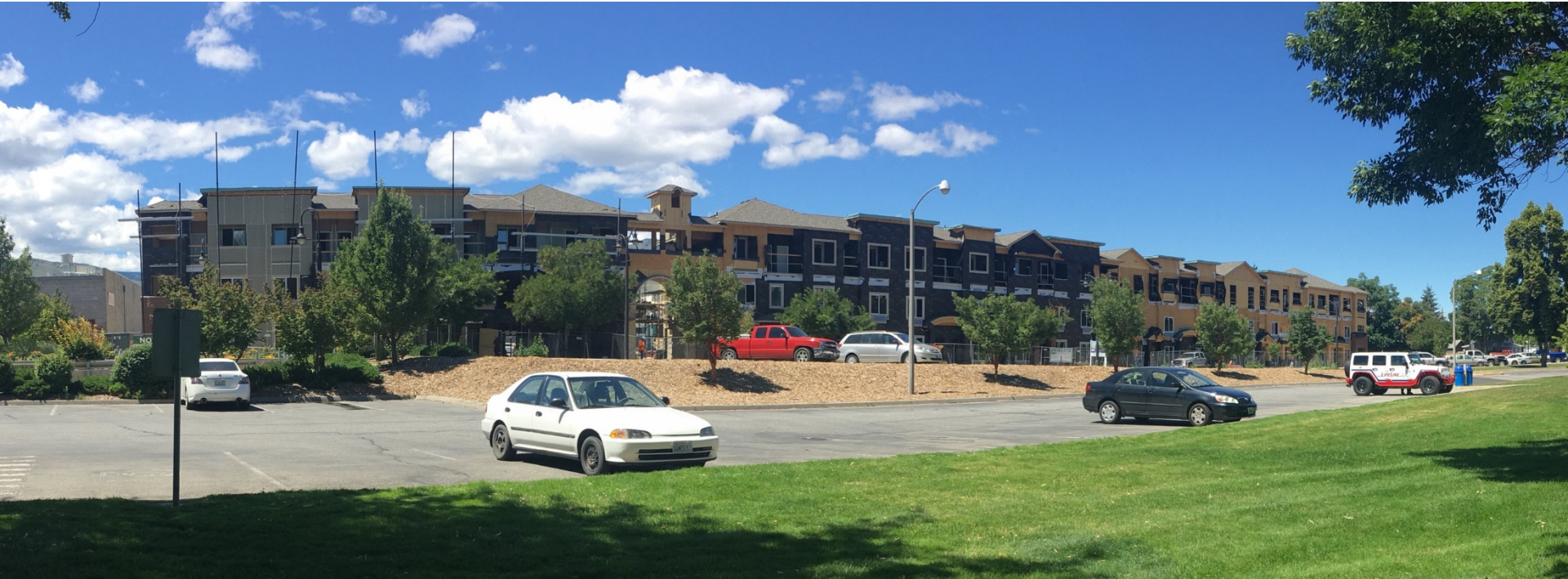
Photo: Riverside Drive Apartments- Wenatchee
