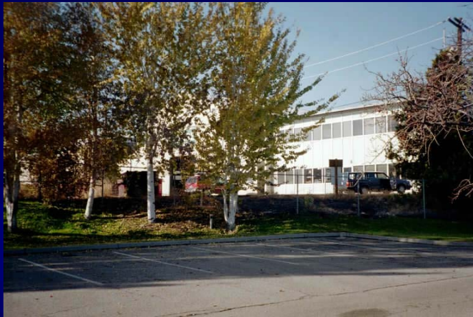
Existing frontage on Orondo
