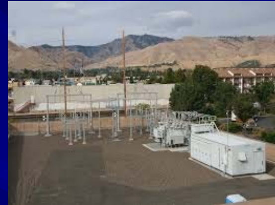
Utilities Walla Walla Substation
