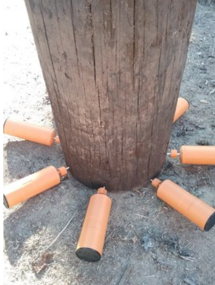
Non-destructive Ultrasonic Pole Inspections
