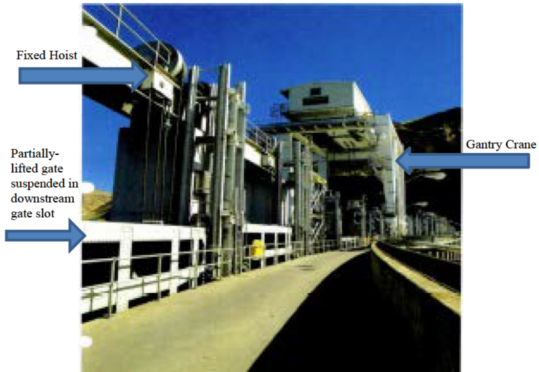
Photo No. 1 - View of spillway bays along spillway deck. The spillway bay in foreground is outfitted with a fixed hoist while a gantry crane is positioned over bay/gate in background.
