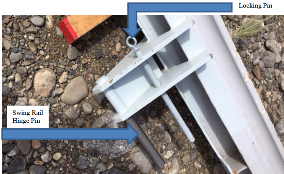
Photo No. 4 - Gate 17's north swing rail lower hinge assembly with hinge pin (left) and locking pin (right). The swing rail was removed from the spillway after the incident and relocated to a maintenance yard adjacent to the Dam.
