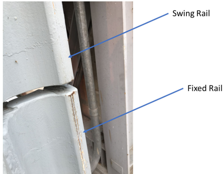
Photo 6; Gate 17 South Stanchion –Gap and Slight Misalignment Between Fixed Rail and Swing Rail
