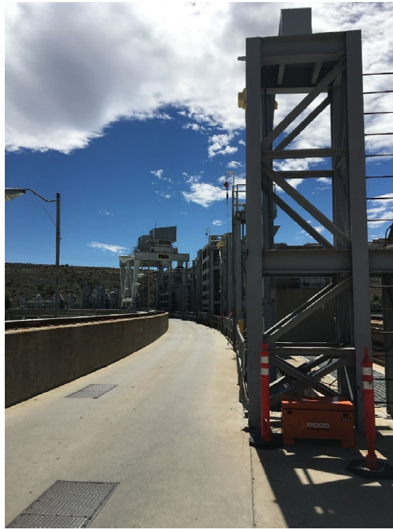
Photo 1: Rock Island Dam Deck Supports Multiple Stanchions for Removal and Storage of Segmented Lift Gates
