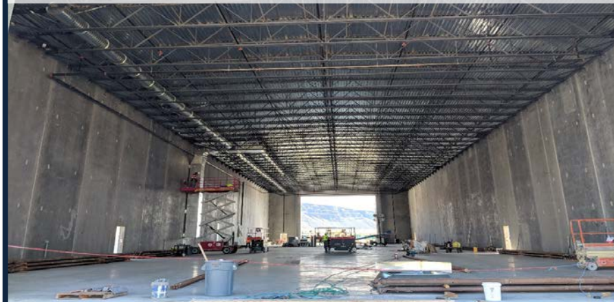
RI and RR facilities upgrades
