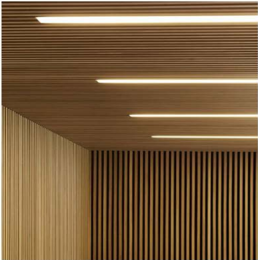
EXAMPLE(S) OF NATURAL WOOD SLAT WALL SURFACES AT CEILINGS AND SELECTED WALLS
