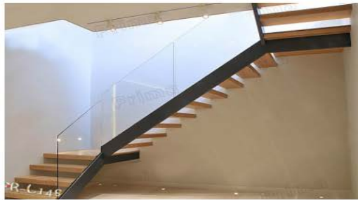
EXAMPLE(S) OF STEEL STAIR W. WOOD TREADS, FRAMELESS GLASS RAIL W./ALUM. HANDRAIL
