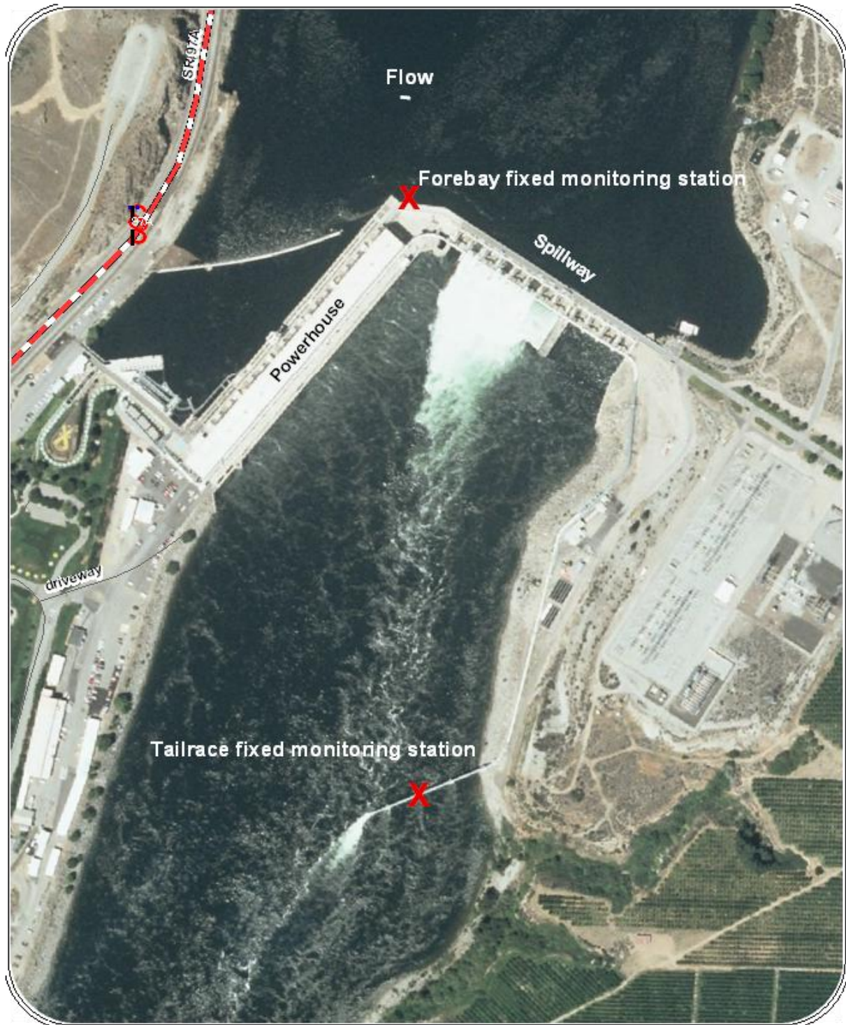
Figure 5-1: Locations of the Forebay and Tailrace Fixed Monitoring Stations at Rocky Reach.
