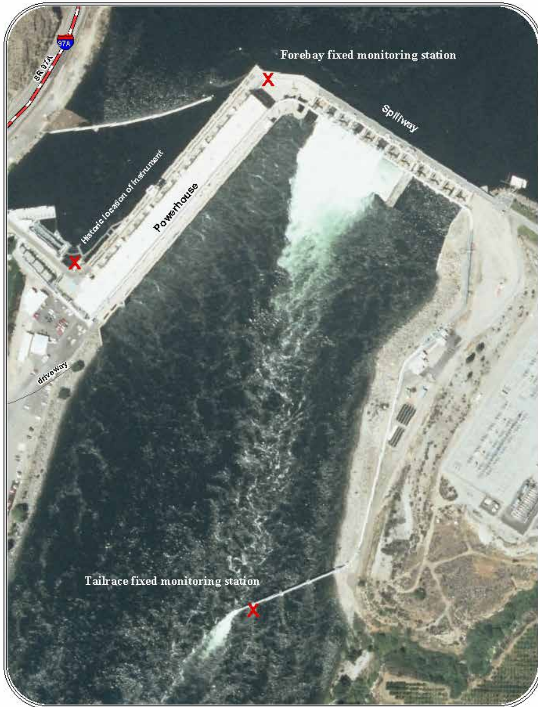
Figure 1-2. Rocky Reach Dam forebay and tailrace fixed monitoring stations
