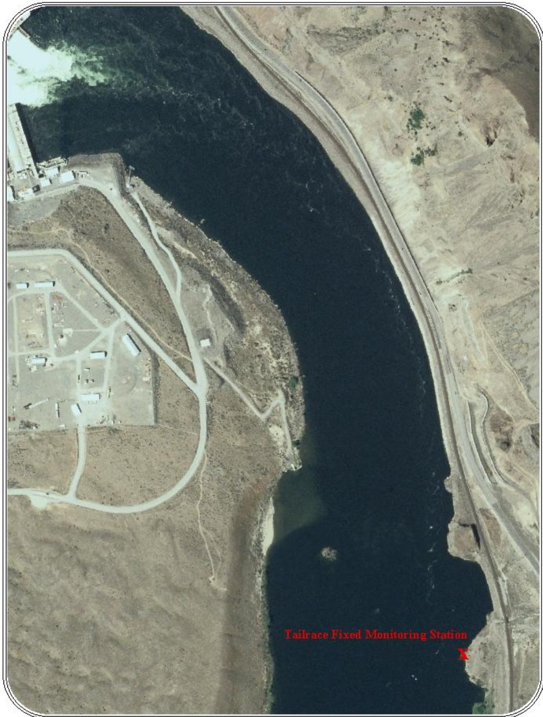
Figure 2-4: Rock Island Dam, tailrace fixed monitoring station.
