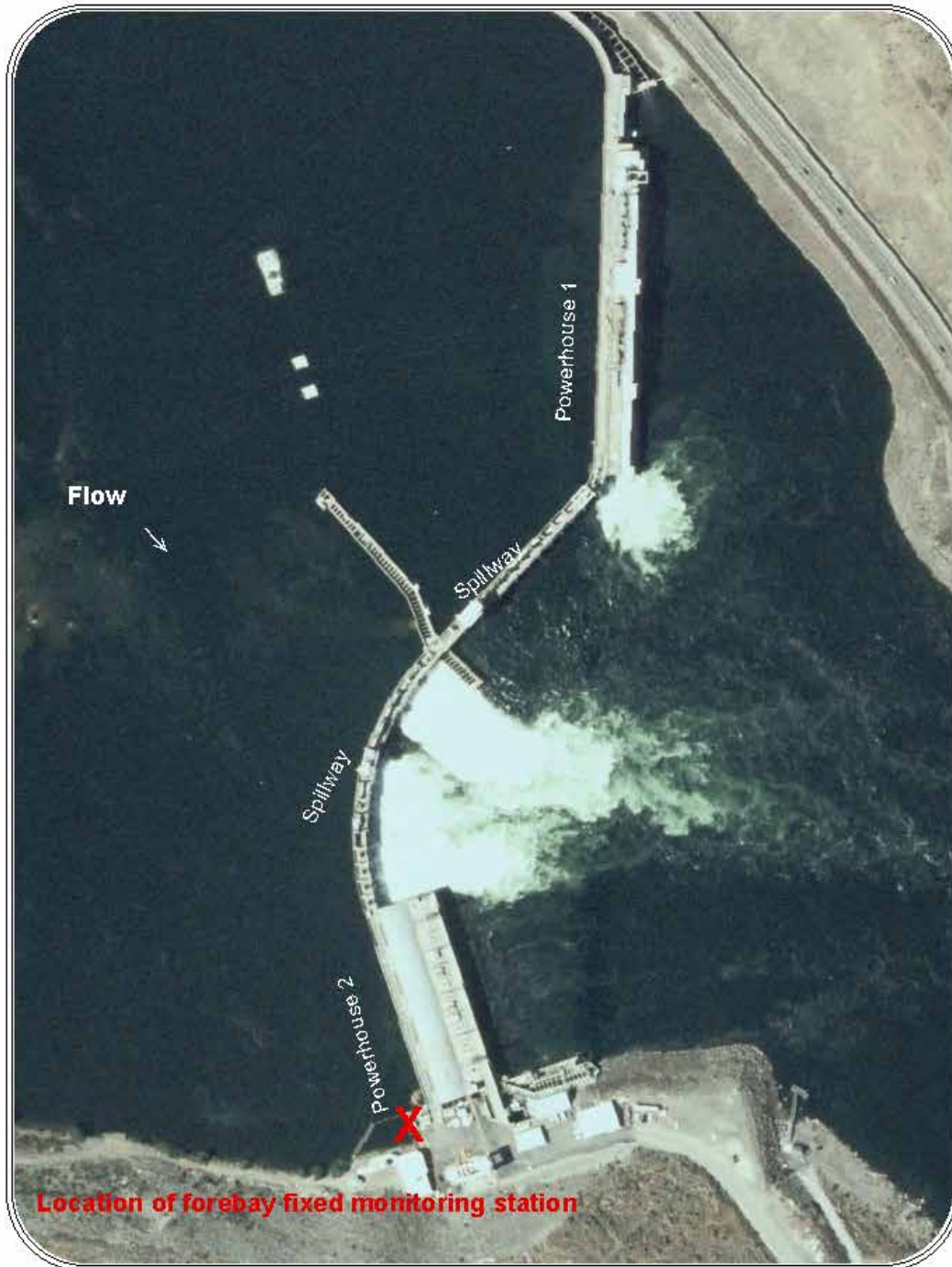
Figure 1-3. Rock Island Dam forebay fixed monitoring station
