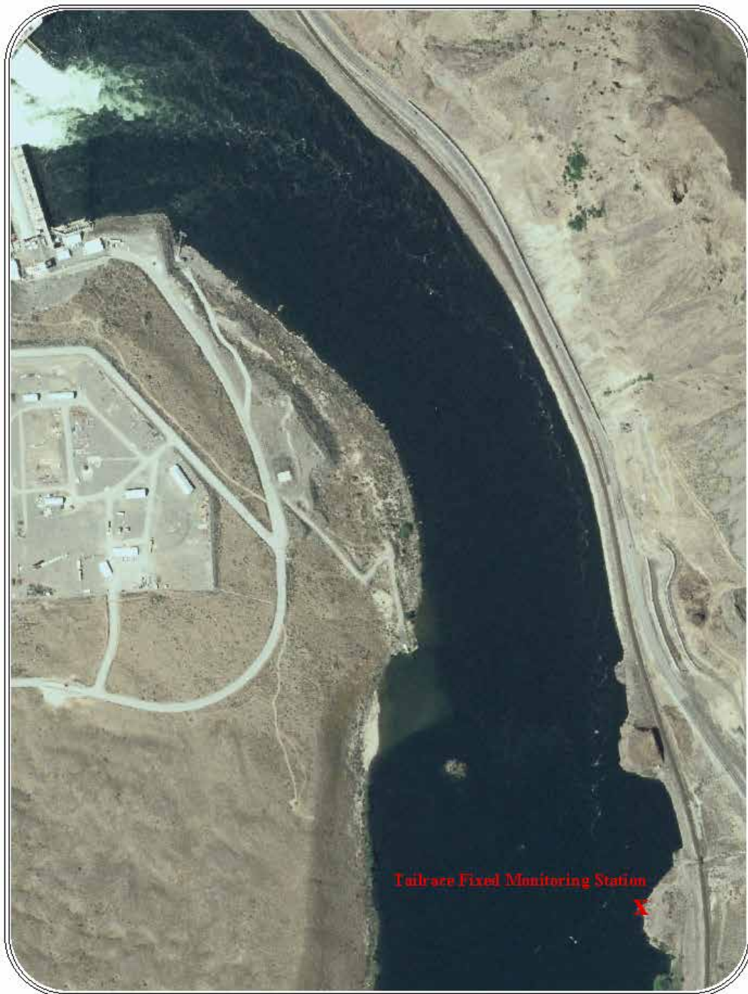
Figure 1-4. Rock Island Dam tailrace fixed monitoring station
