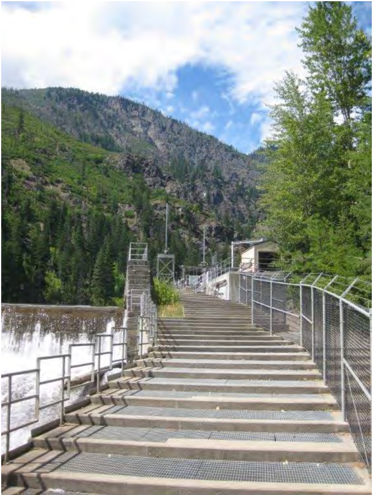
Figure 2. Left Abutment and Fishway Chelan PUD Tumwater Fishway Modifications
