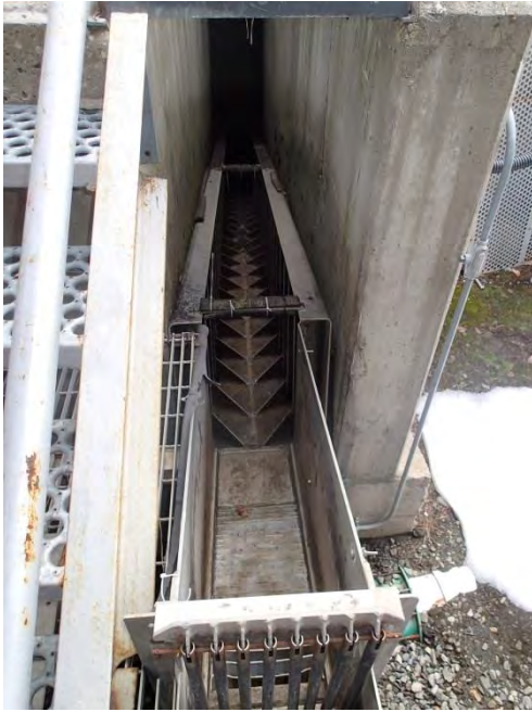
Figure 25 – False weir at top of steep-pass
