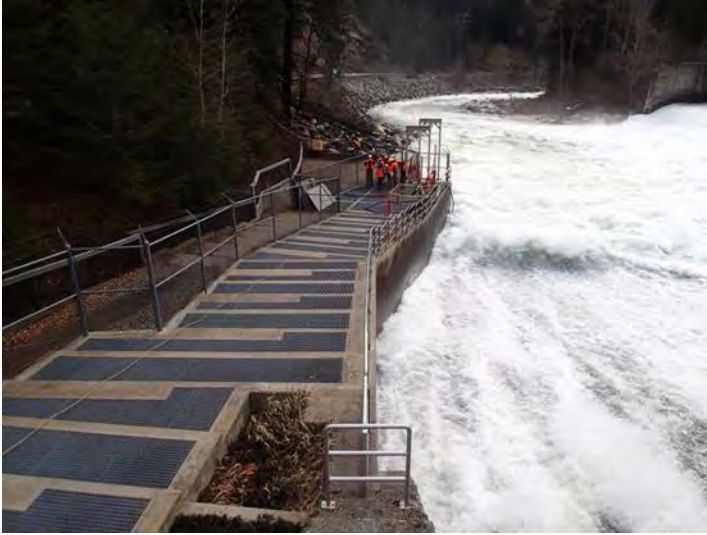
Figures 5 and 6. Turbulent tailwater adjacent to fishway on day of site visit
