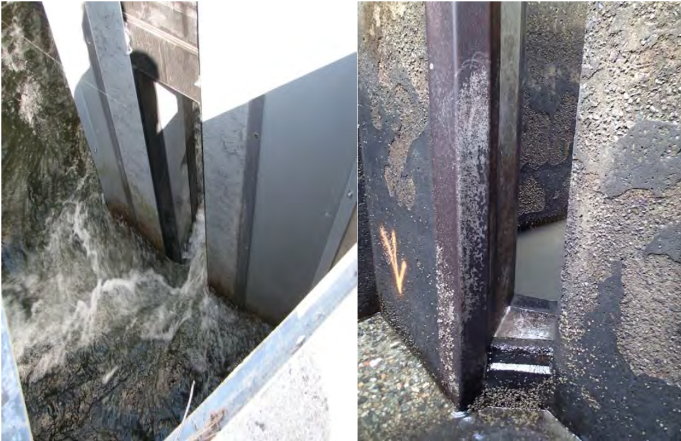
Figure 17 and 18. PIT detectors with short-channel flow at Slots 15 and 18
