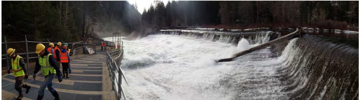
Figure 3. February 18, 2015 site visit tailrace hydraulic conditions at 4380 cfs (Peshastin gage)
