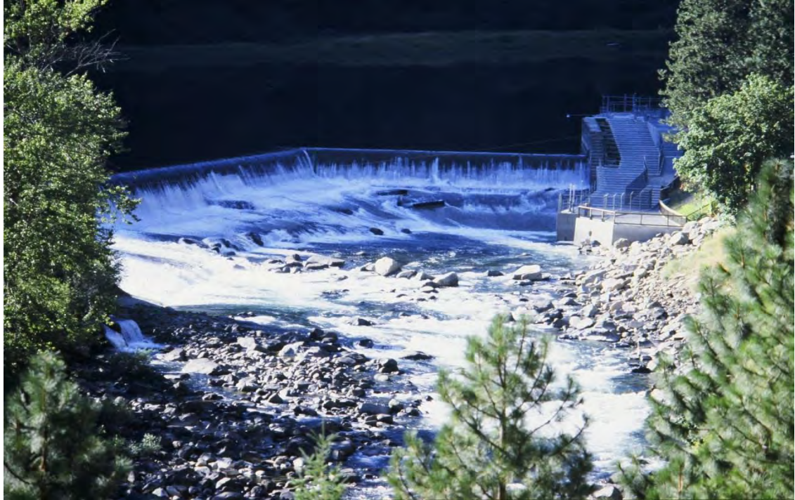
Figure 4. Dam Dog-leg Jet (jet extends diagonally to left shore near the fishway). Note that this is a previous photo during relatively low discharge period
