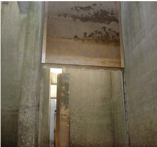
Figure 22 – Closure bulkhead to initiate trapping operations, at Weir 19
