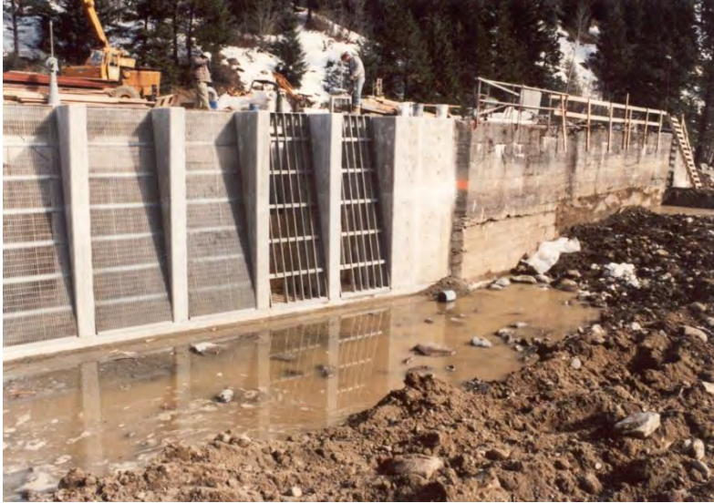
Figure 19. Tumwater AWS and lower ladder trash racks
