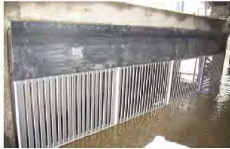
Reduced access to area behind count station crowder
