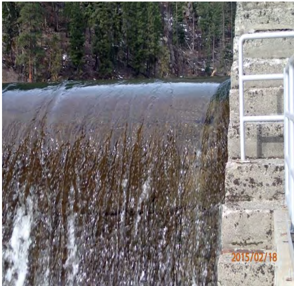
Figure 26 – Flow over dam ogee
