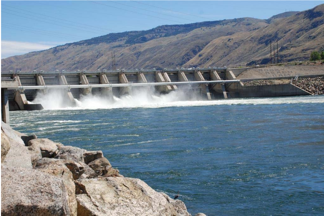
Figure 3. Rocky Reach Project spillways.
