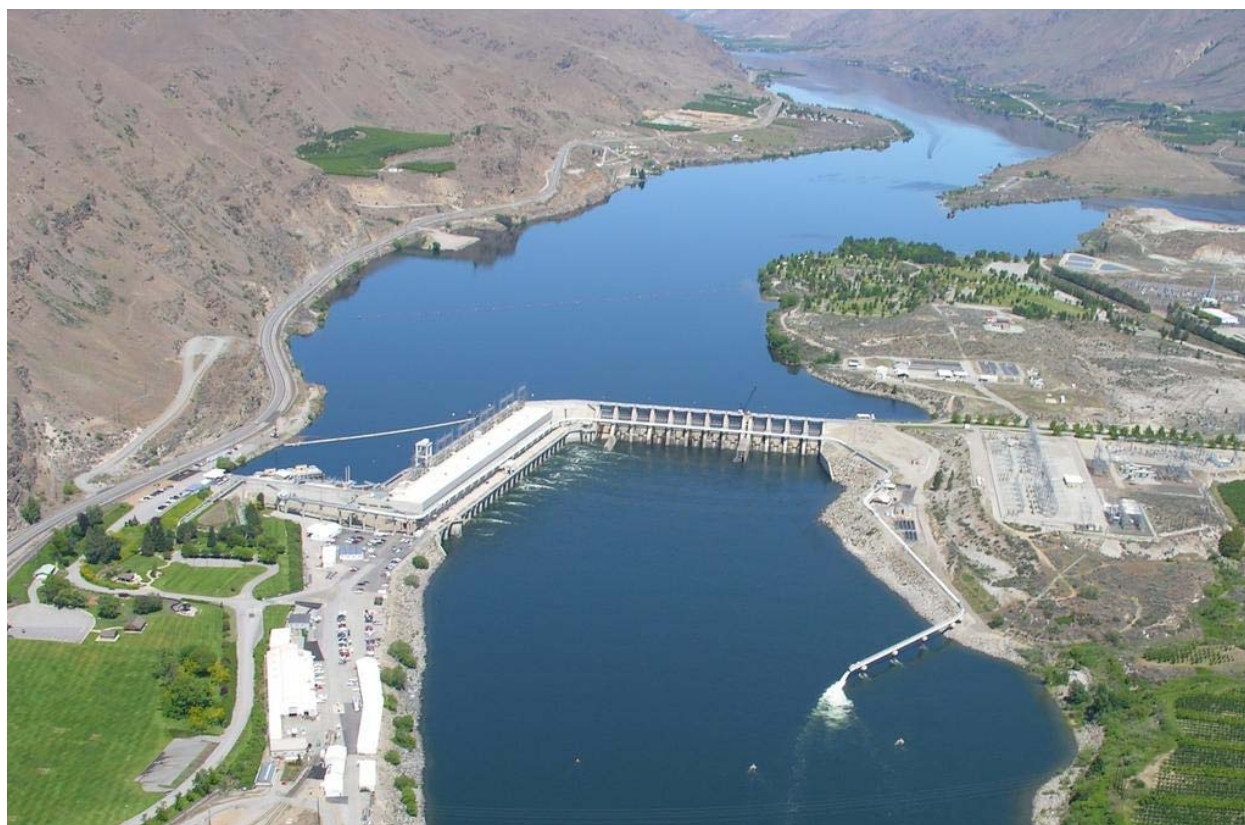
Figure 2. Rocky Reach Dam.
