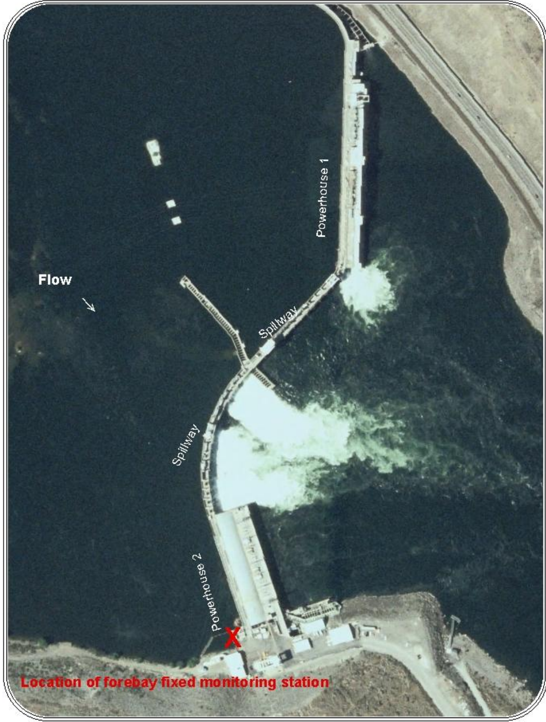
Figure 2-3: Rock Island Dam, forebay fixed monitoring station.
