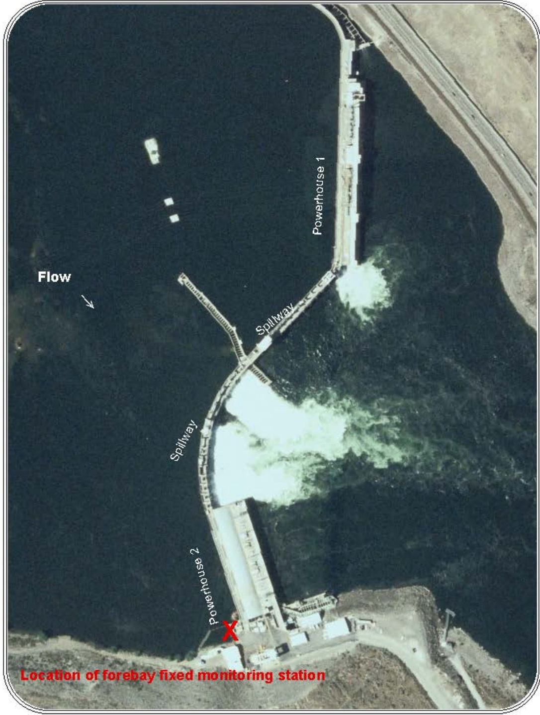
Figure 2-3: Rock Island Dam, forebay fixed monitoring station.
