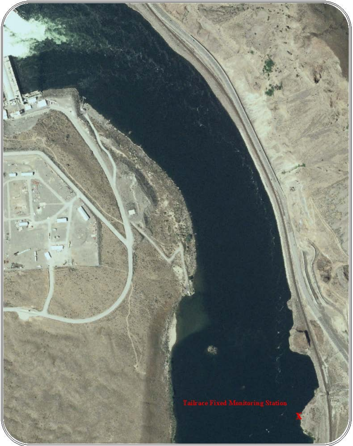
Figure 3-2: Location of tailrace fixed monitoring station below Rock Island Hydroelectric Project.
