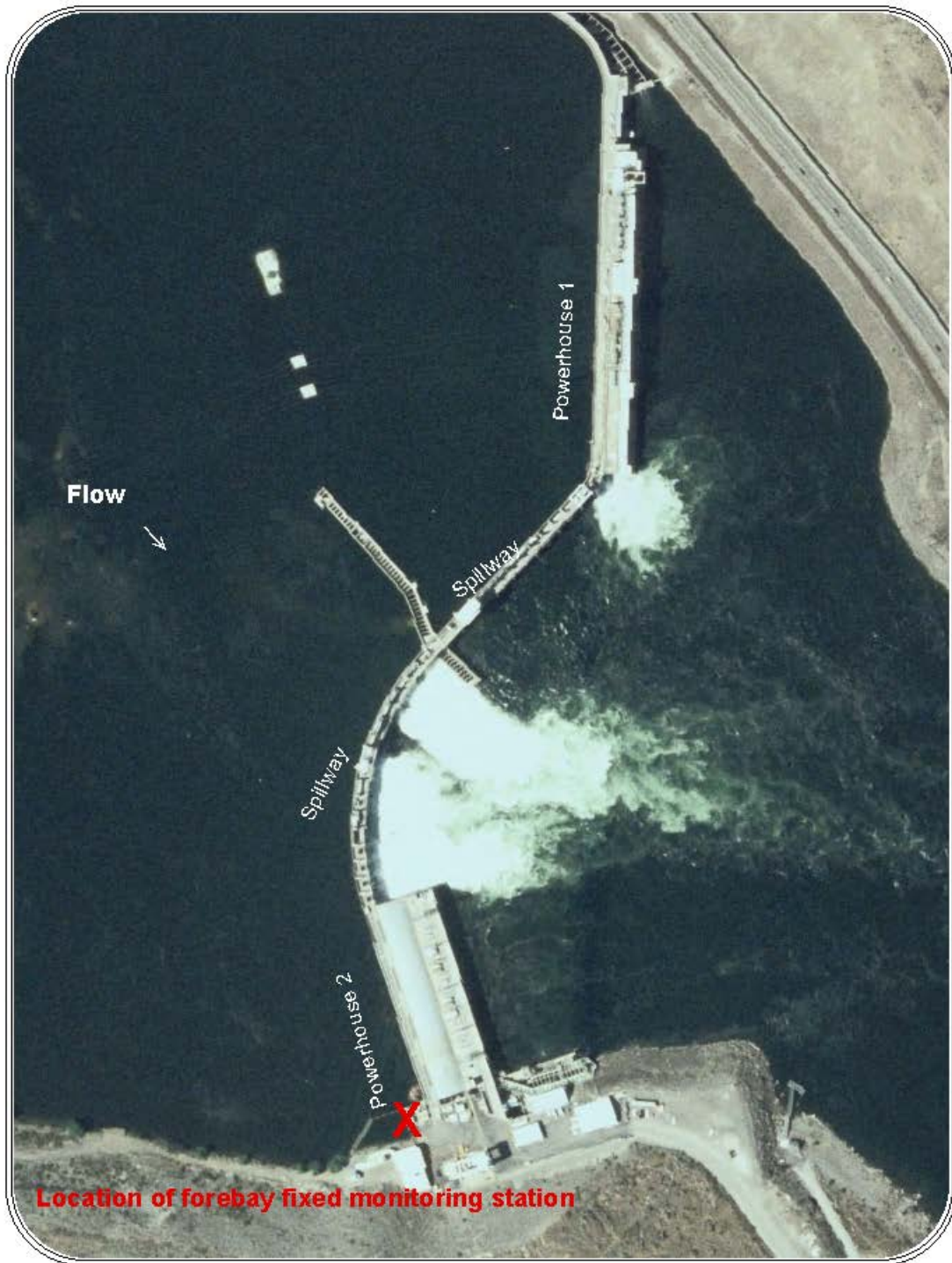
Figure 2-3: Rock Island Dam, forebay fixed monitoring station.
