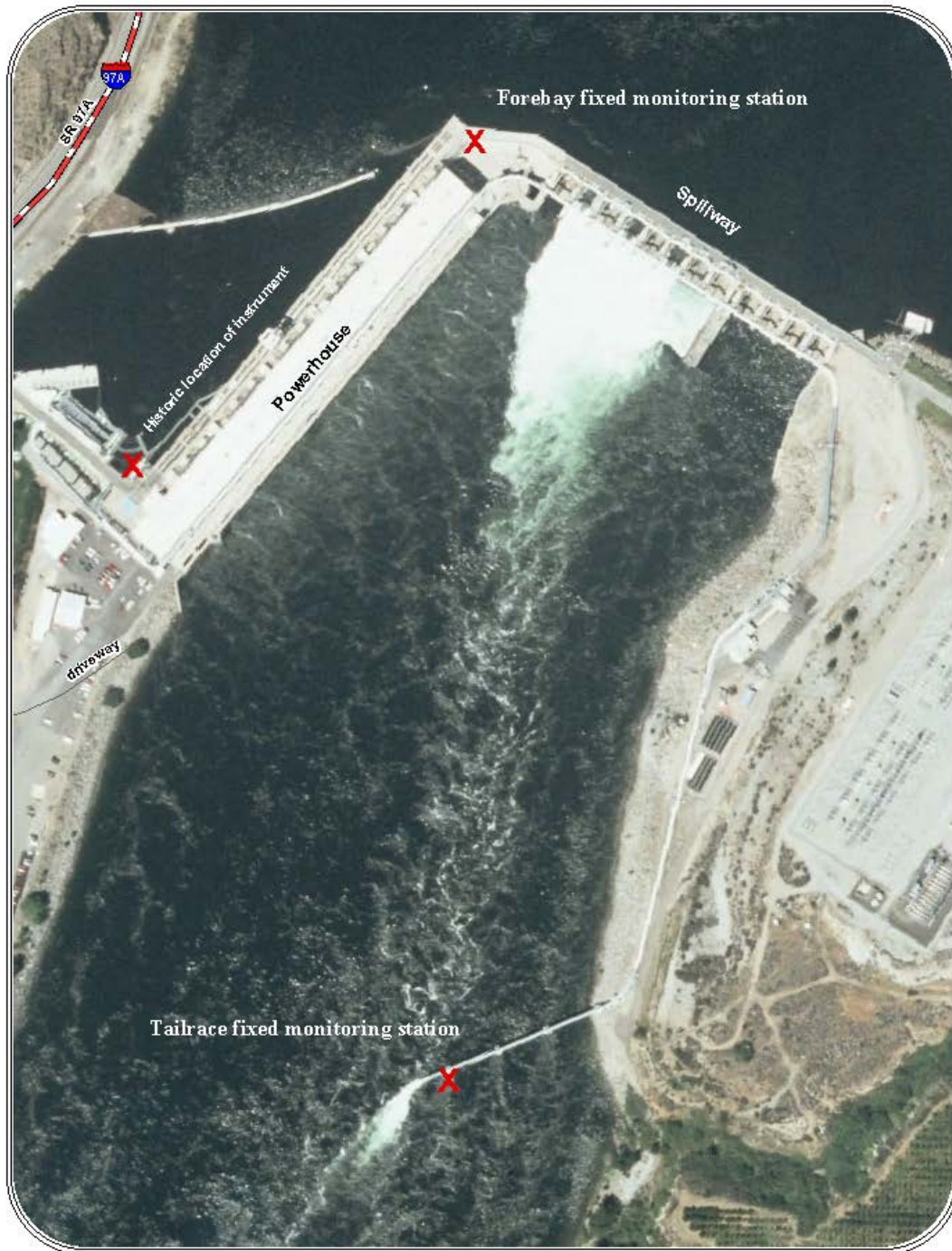
Figure 3-1: Location of forebay fixed monitoring station at Rocky Reach Hydroelectric Project.
