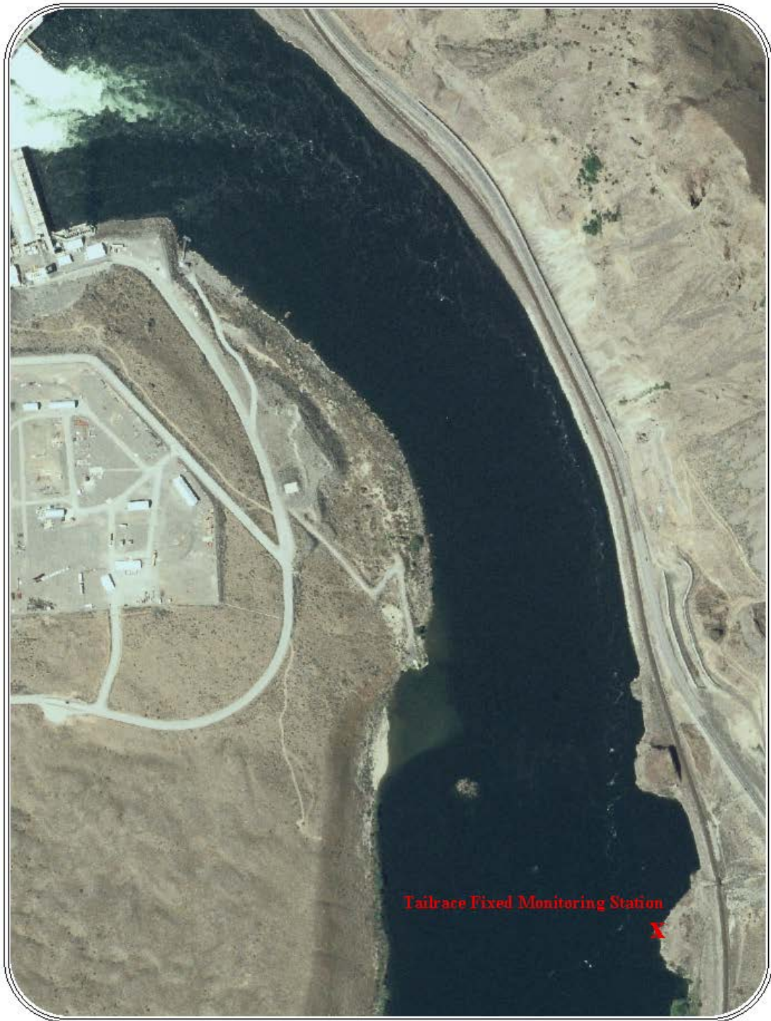
Figure 2-4: Rock Island Dam, tailrace fixed monitoring station.
